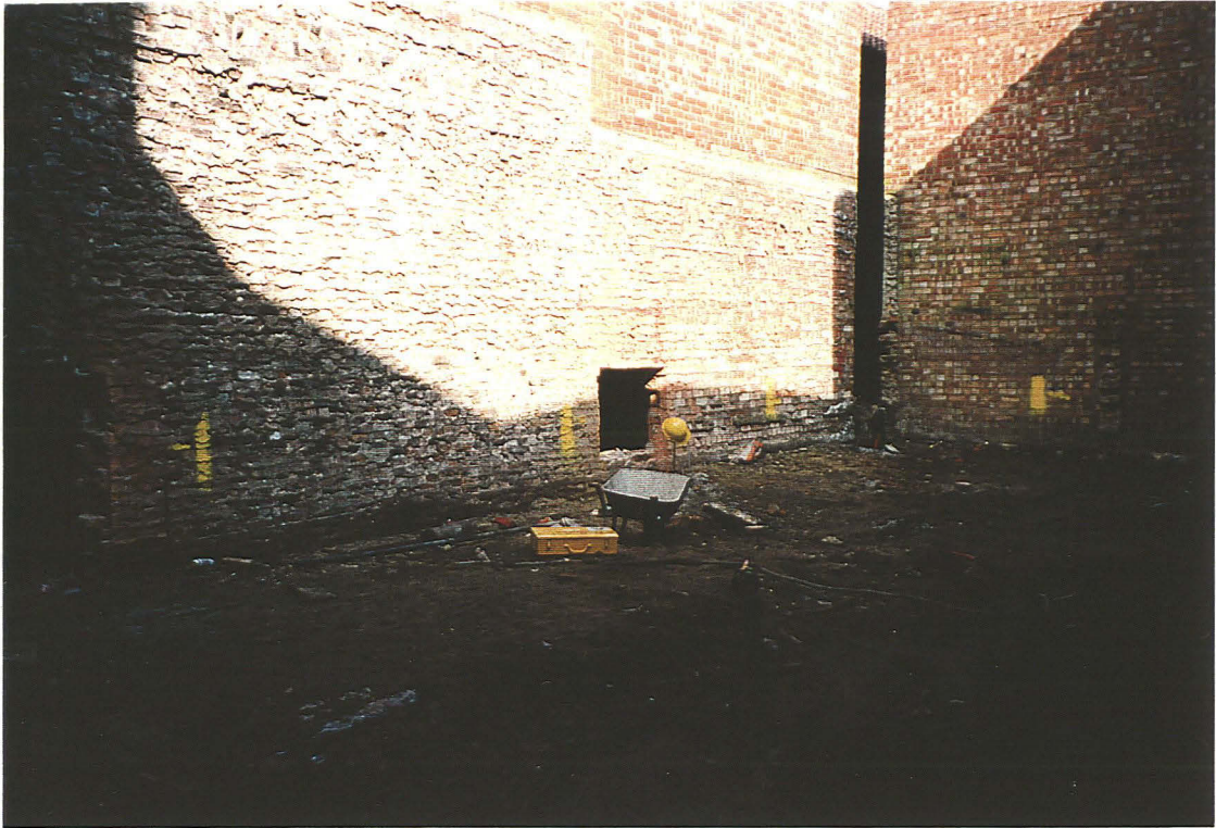
P.1 General view of the yard area, looking north east.
