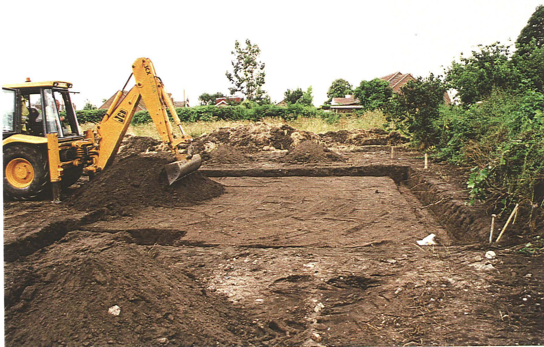
P.2 View of soil stripping for the raft foundation in progress, looking south.
