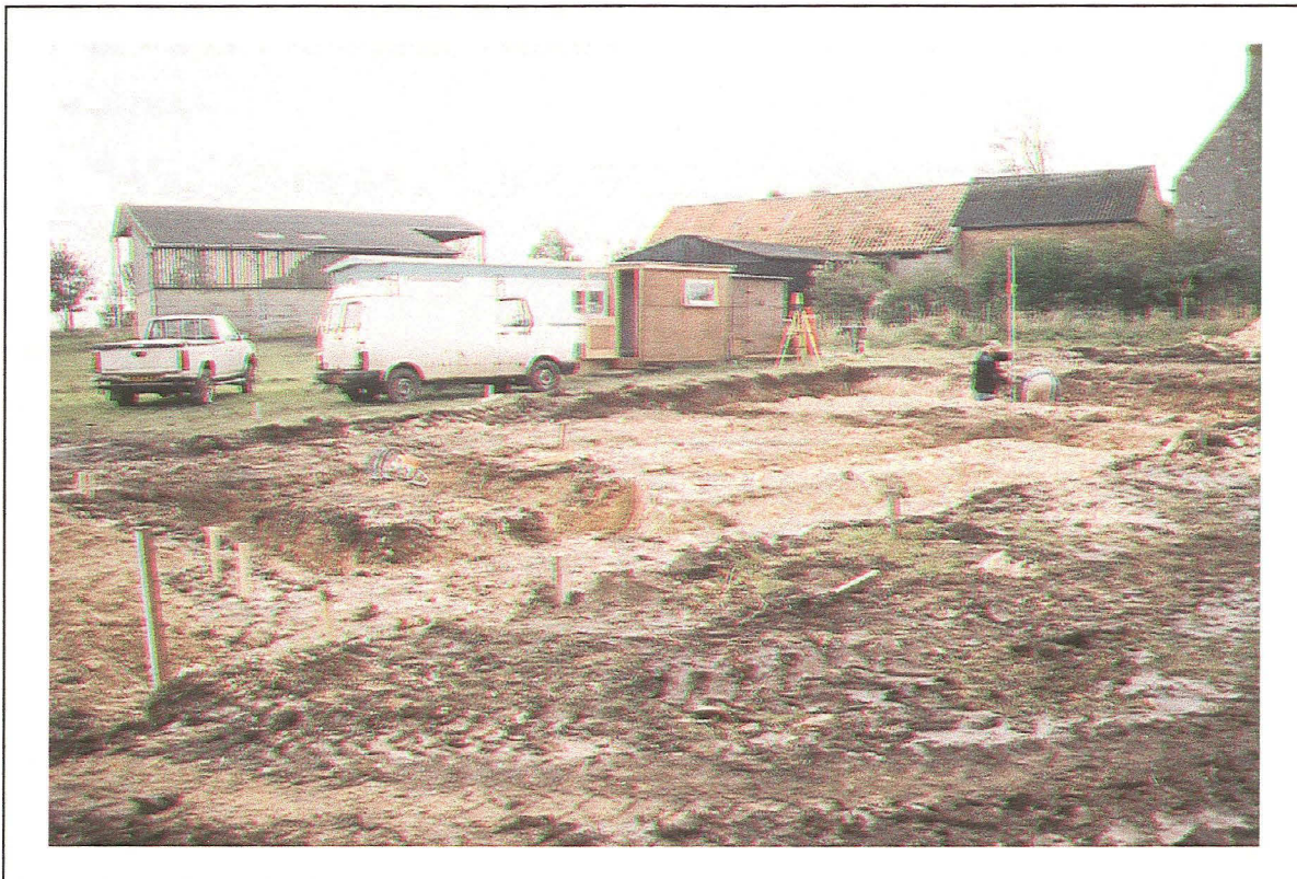
Plate 1: General view of site, following stripping & foundation trenching - looking south-west
