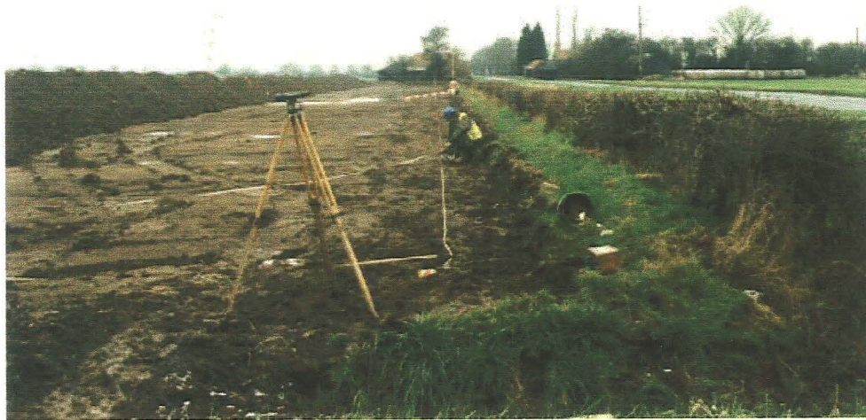
Plate 1 - General view of the excavated area, prior to cleaning, looking north
