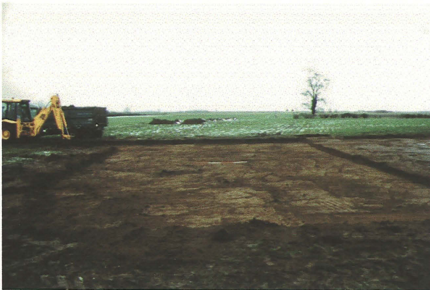
Plate 2 View of stripping, facing N
