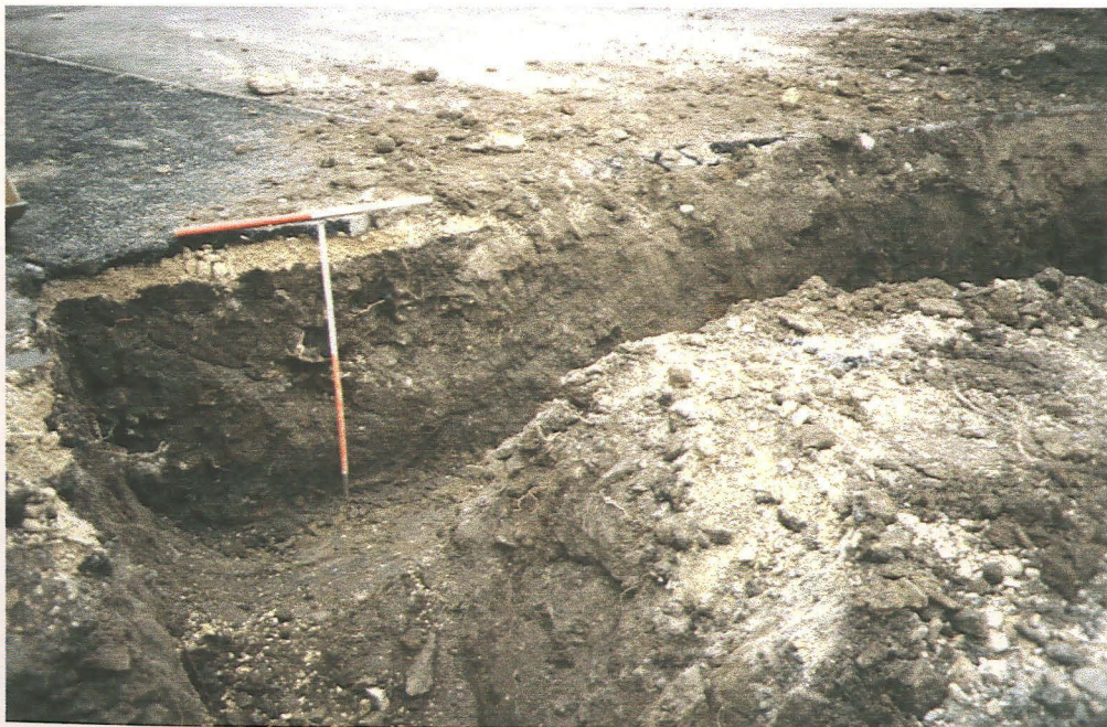
Plate 4 View of made ground (section 4), looking south
