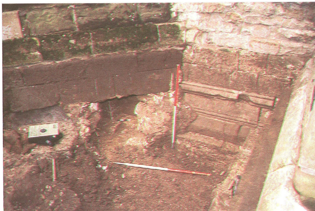
Plate 3: View of original tower corner (and small buttress) exposed beneath existing 1886 buttressing - looking north-west
