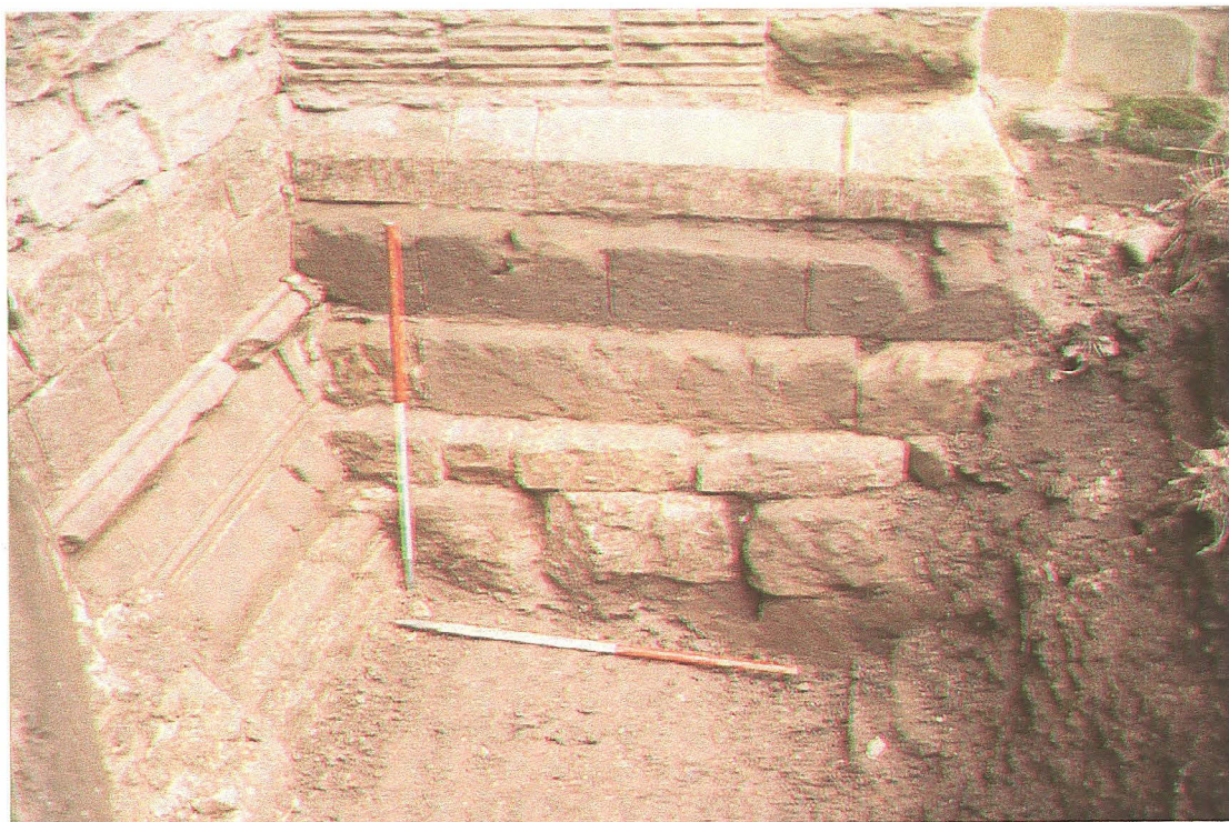
Plate 1: View of exposed foundations of 15 th century buttress (west end of aisle/south side of tower) - looking east
