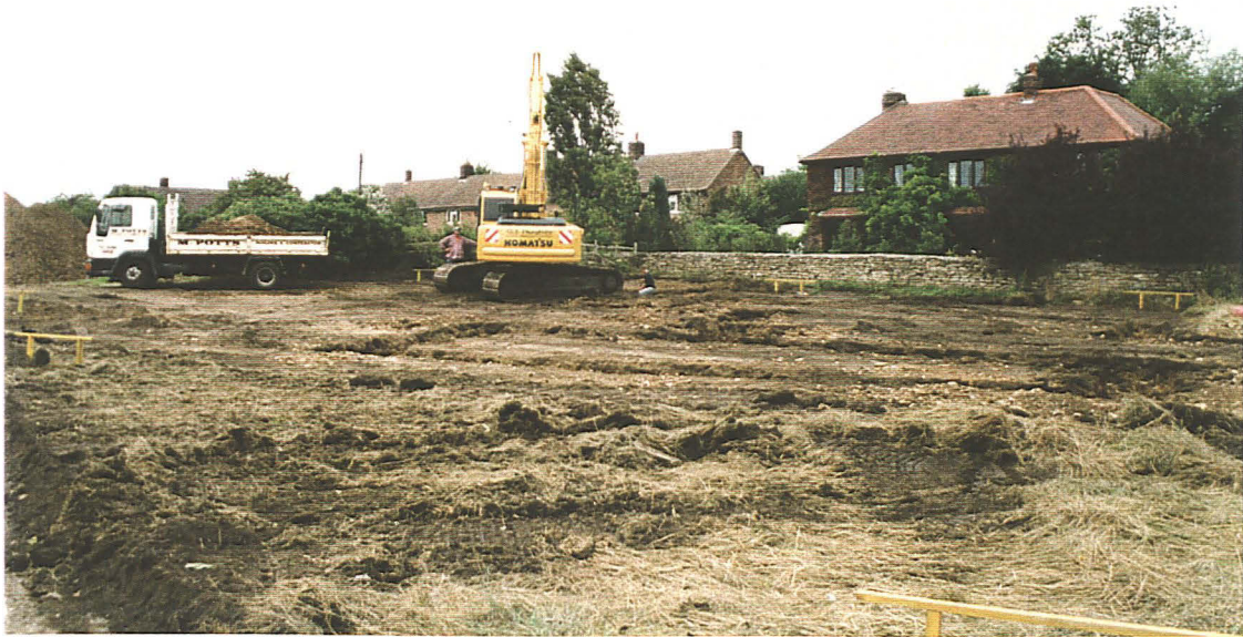
P.3 General view of Plot 2, looking north-west.
