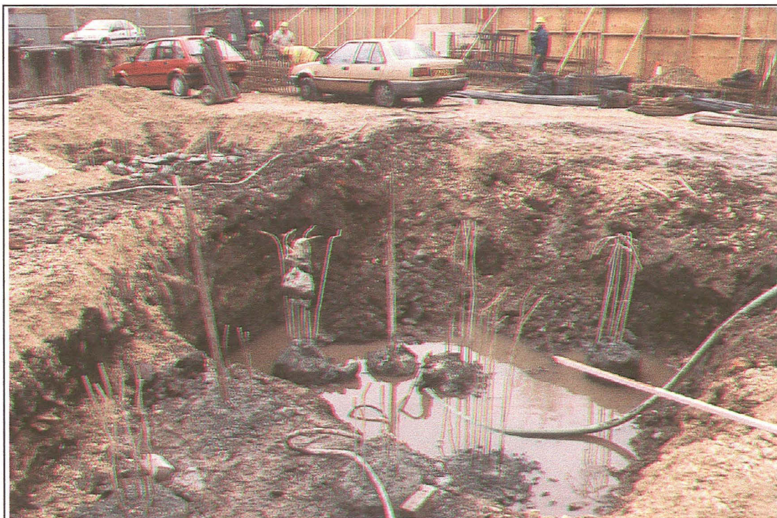
Plate II: General view of the lift pit trench looking south-east.
