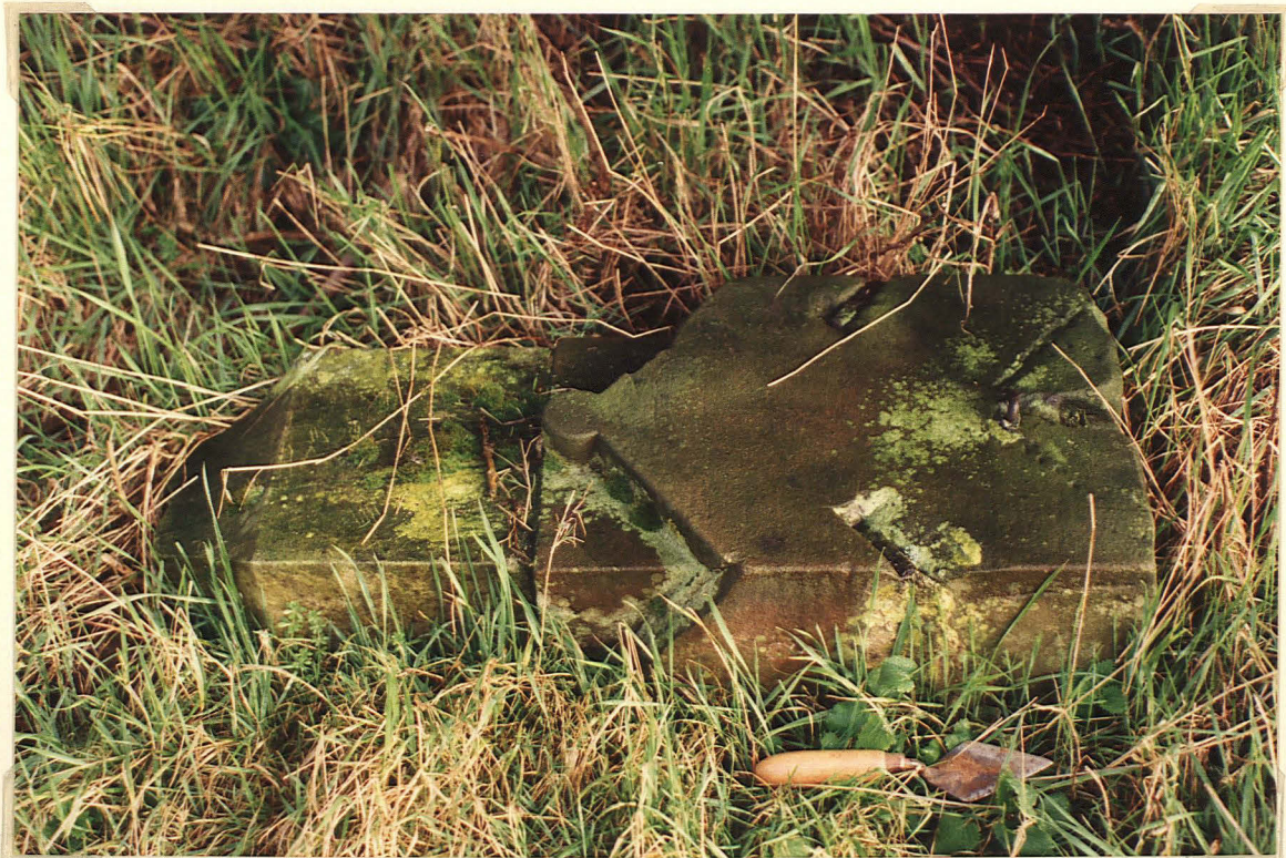
6 Methodist chapel, fallen gate post
