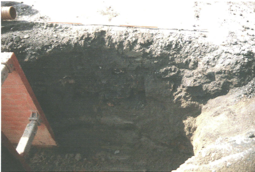
Plate 4 Section 2, showing Service Trench [034] and Soakway [012]
