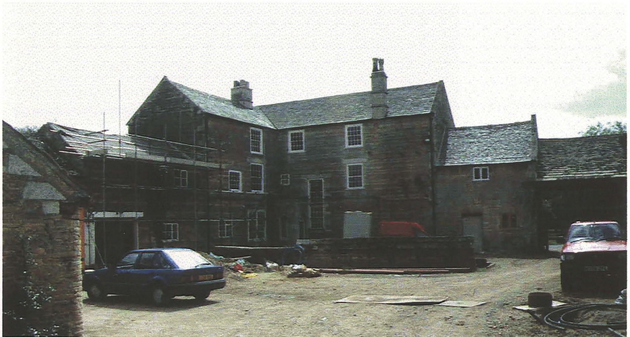
Plate 2 View of Towngate Farm, looking East from front courtyard
