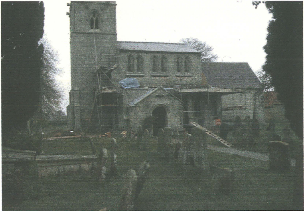
Plate 1 - St Andrew's Church, from the south
