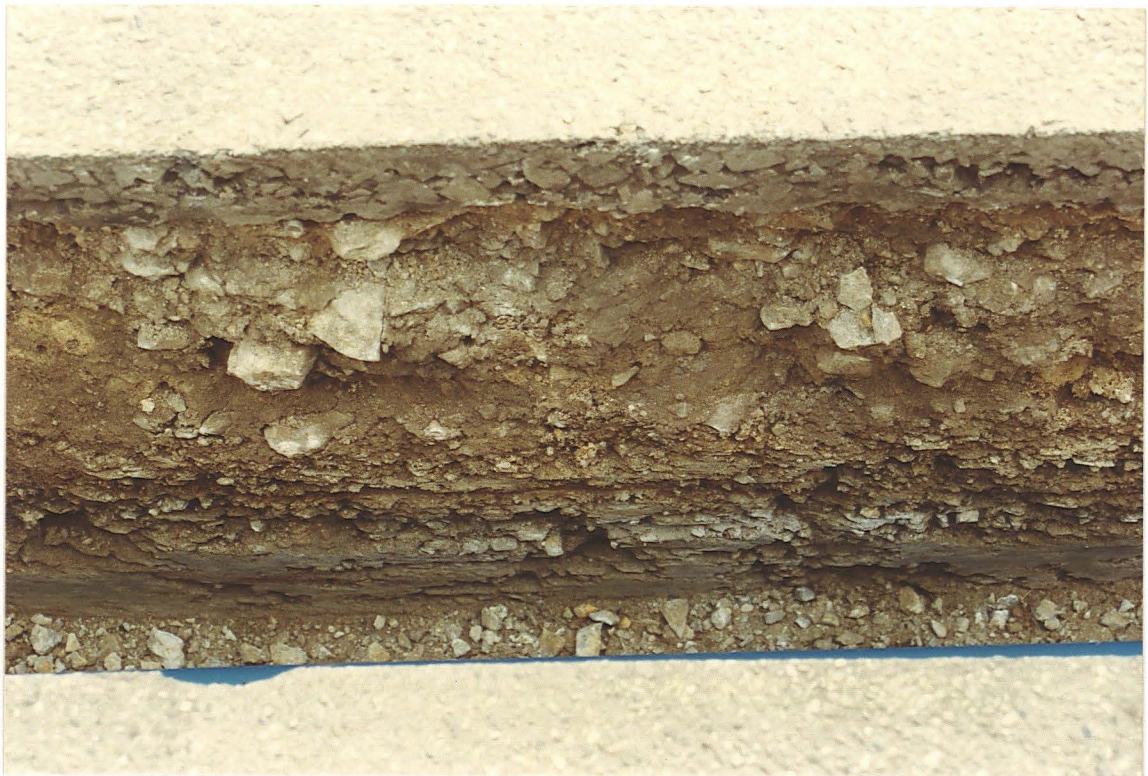
Pl. 4 Bedrock and natural horizontal strata 3 at trench base.
