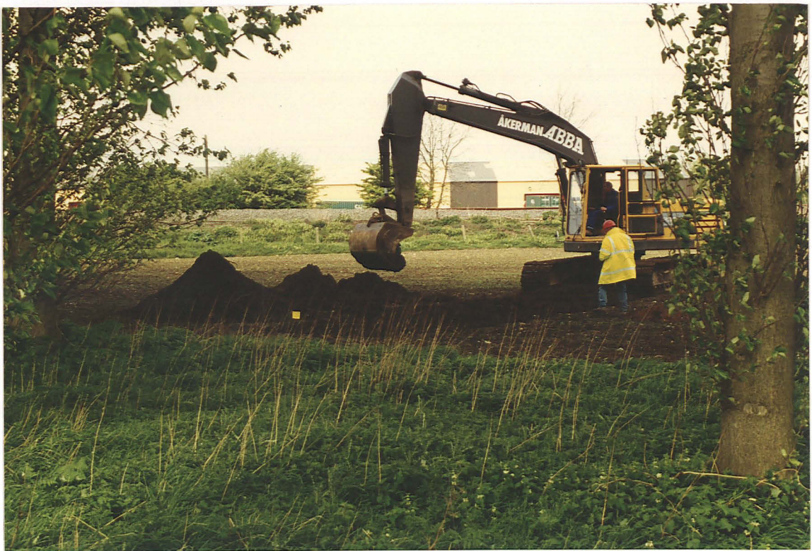
Pl. 3 Machine trenching in Area 2.
