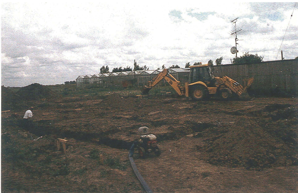
Plate 2: House foundation trenches, general view
