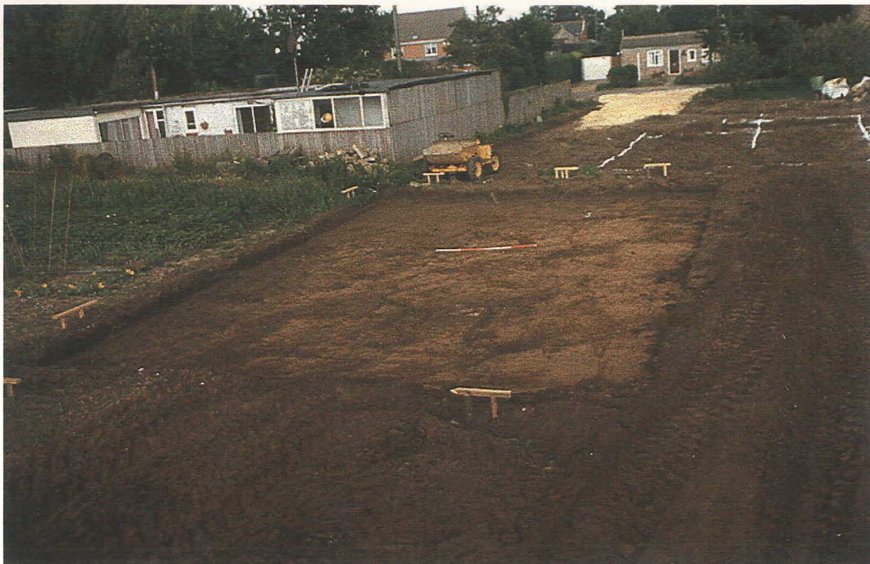
Plate 1: Garage footprint after topsoil stripping
