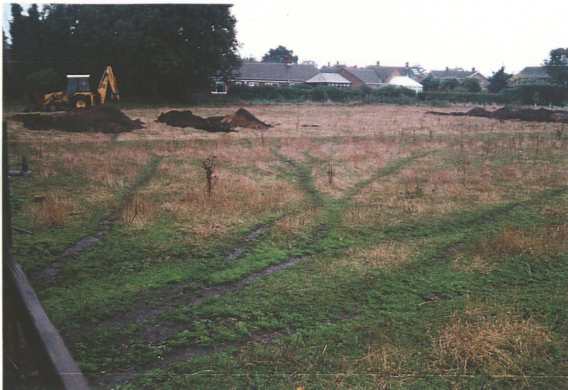
P1. General view of site looking east
