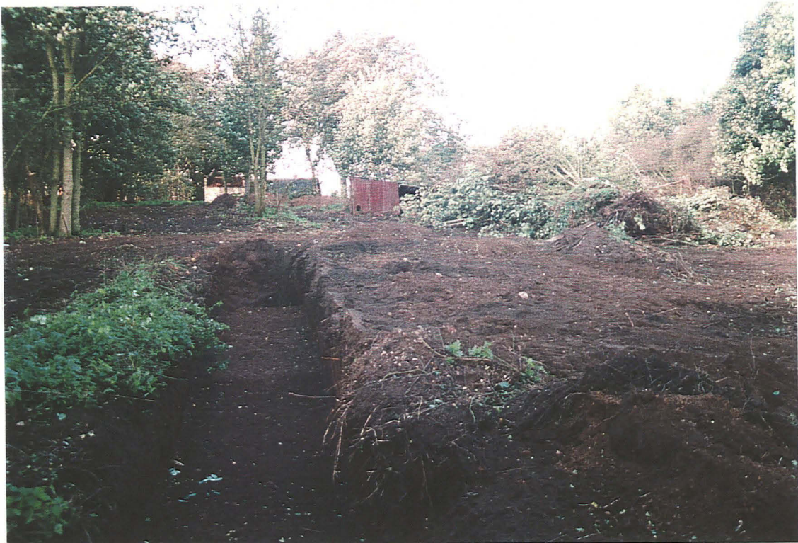
P4. General view of site looking west (Trench 3 in foreground)
