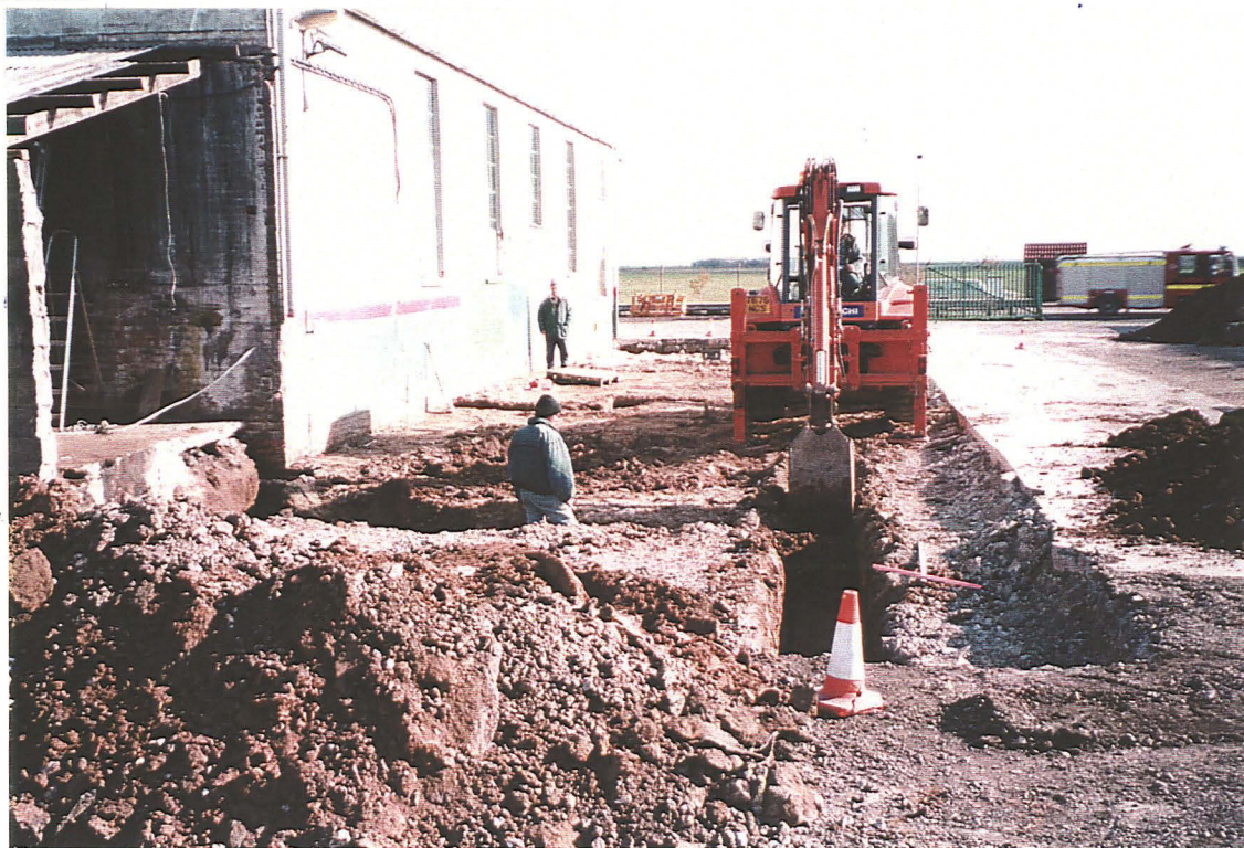
P1. General shot of excavation area during excavation, looking S.E.
