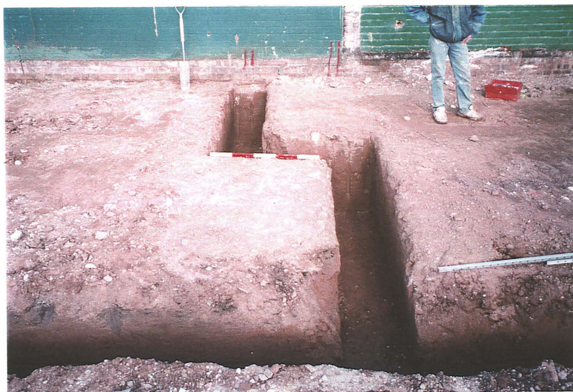
P2. General shot of second foundation trench opened, looking N.E.
