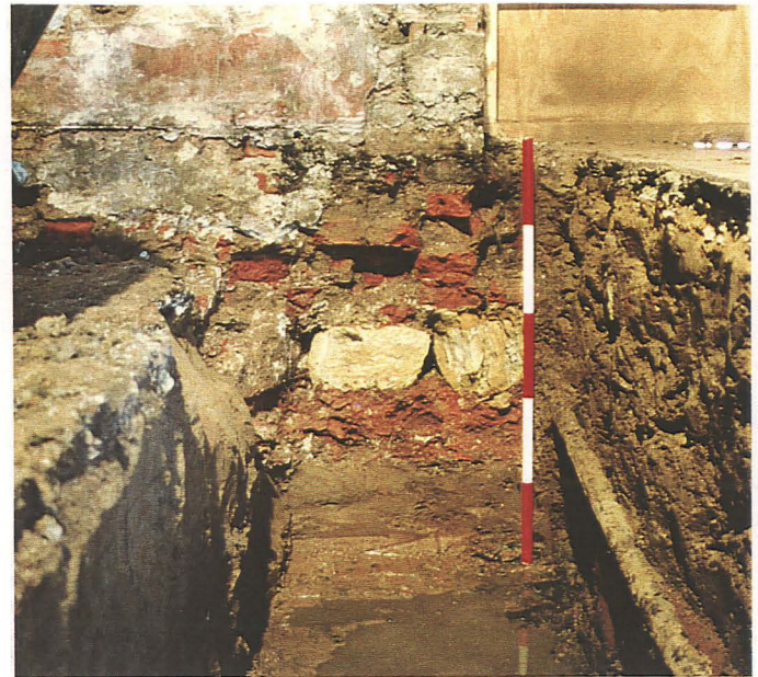
P5. Foundations exposed in north end of east foundation trench (Ref. Fig. 4)
