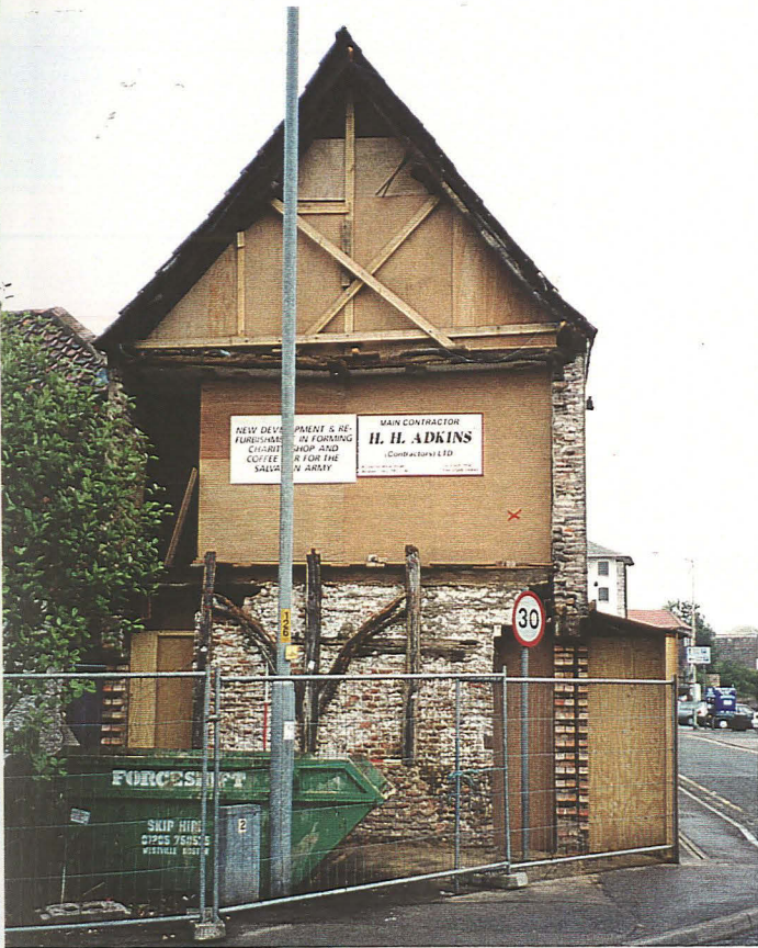
P1. General view of south gable showing exposed timbers
