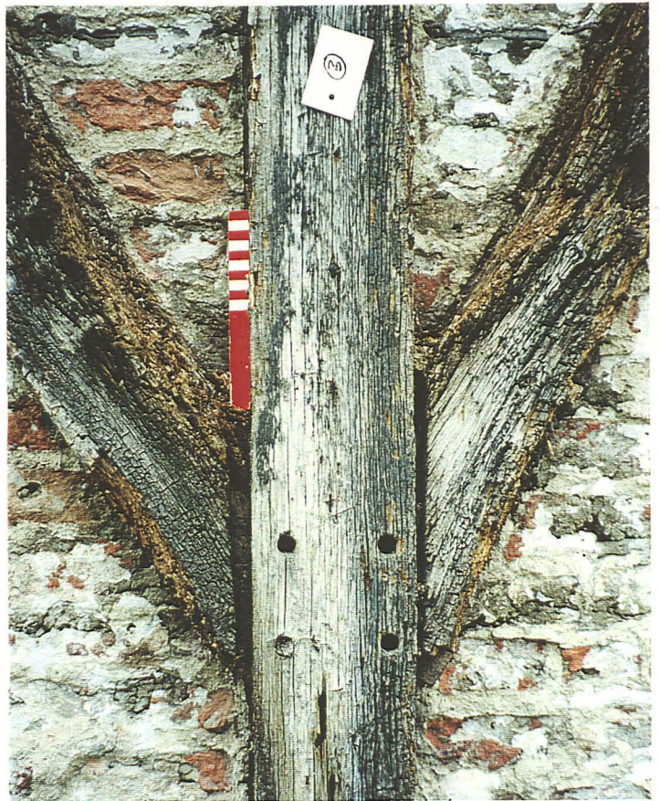
P3. Close-up of timber joints in south gable
