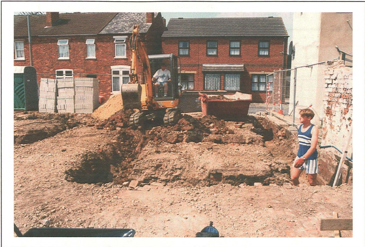
Plate 1: General view of excavation in progress - looking west
