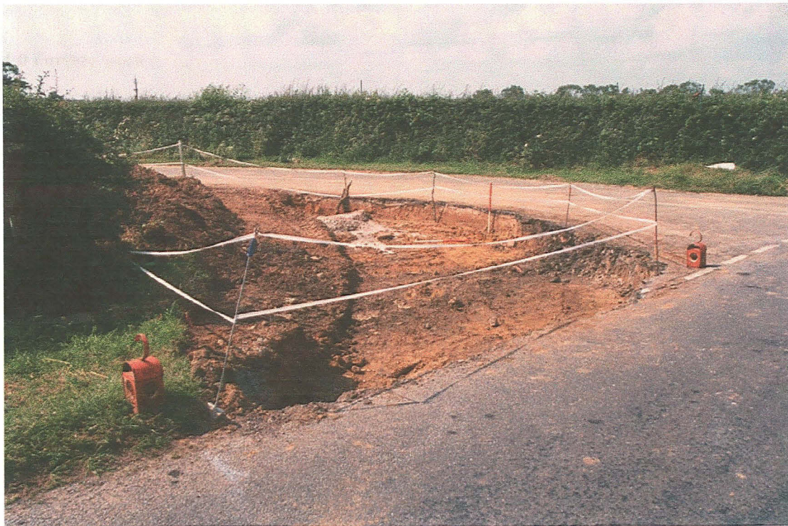
Plate 2: Overall view of modification work to main road junction - looking north-west
