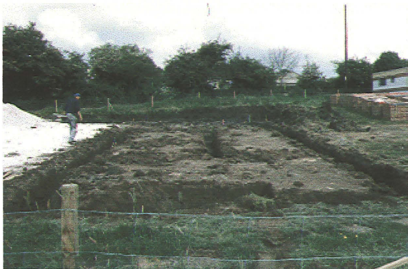
➤ Plate 2 View of foundation trenches
