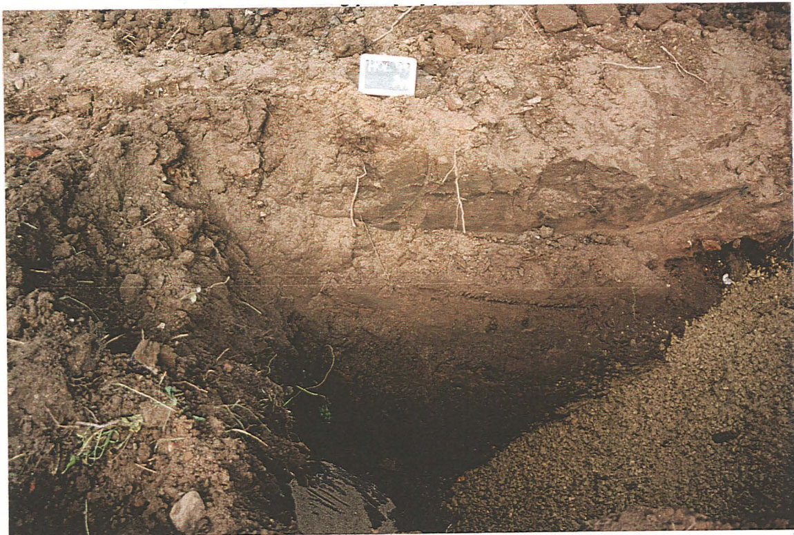
Plate 02: Photograph showing the depth of trenches at Stukely Hall Drive, Holbeach,
