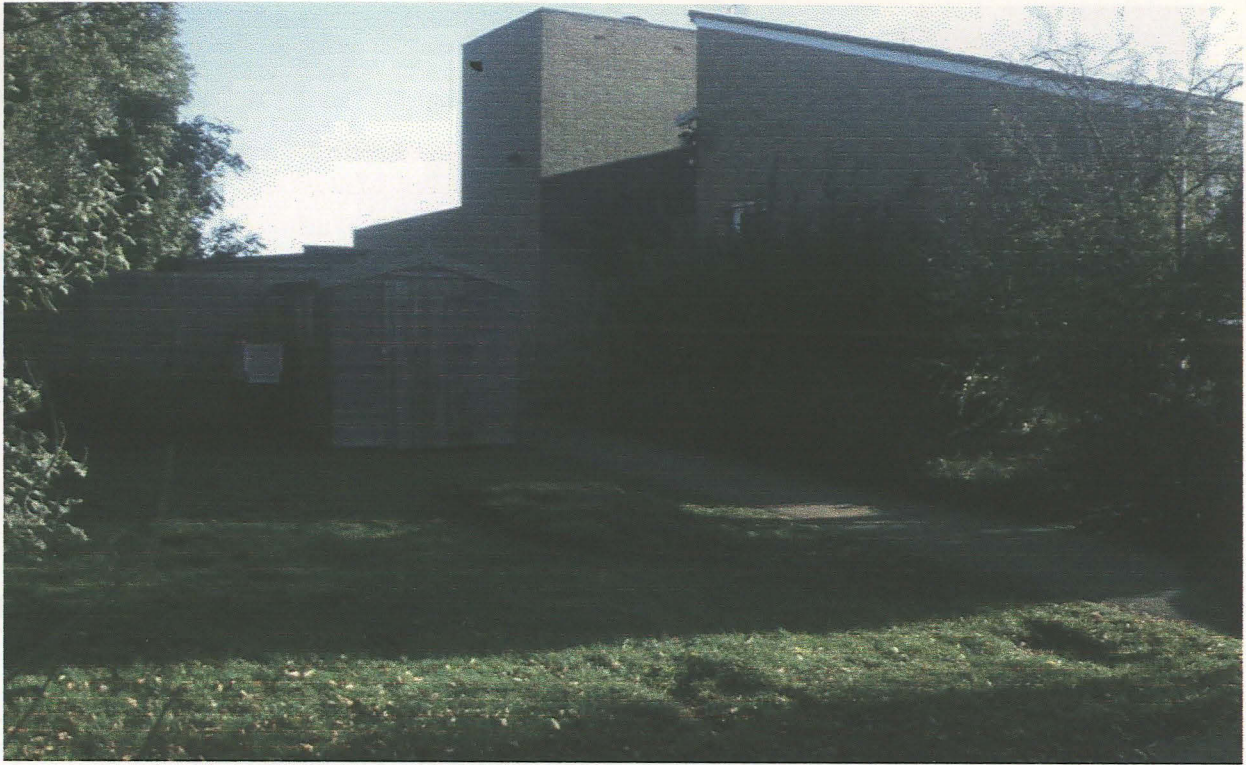
Plate 1 General view of the area of Trench 1
