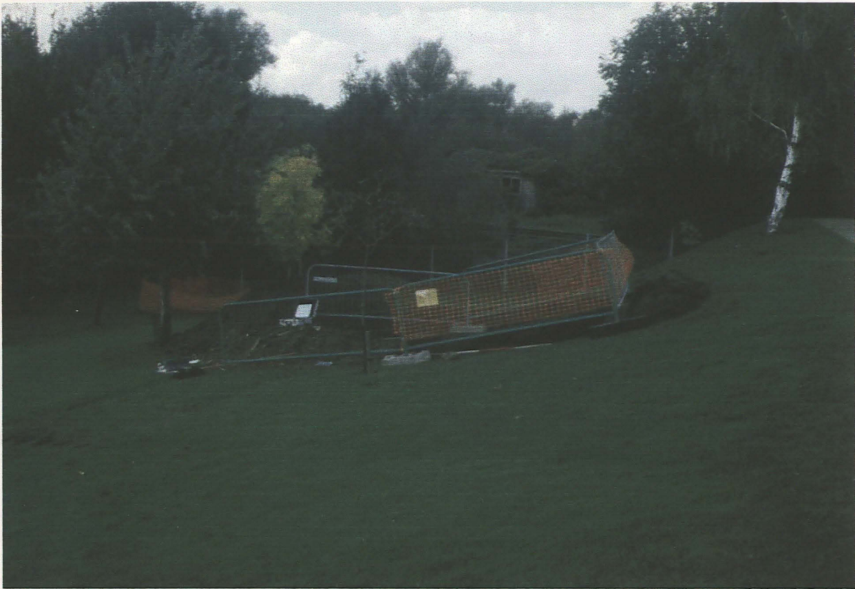
Plate 3 Trench 2, looking north
