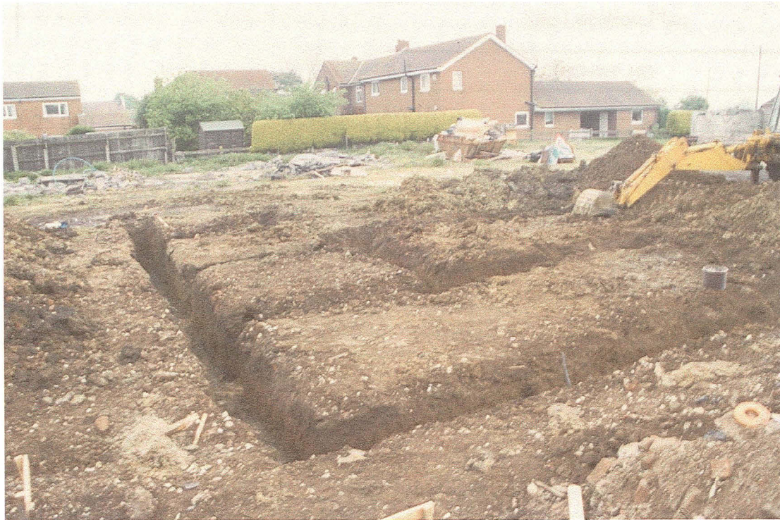
Plate 1: General view of completed foundation trenches, Plot 1 - looking north
