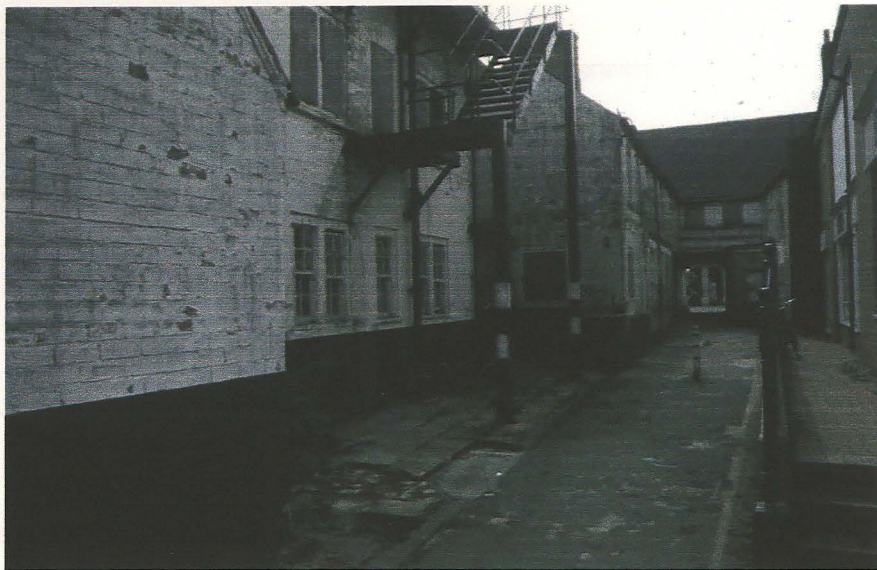
Plate 1 General view of the proposed development area, the Trench is located in the first building in the left
