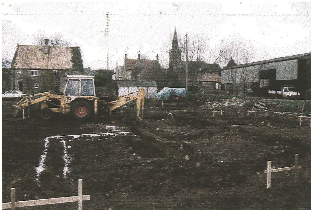
Plate 1 General view of development area, looking north
