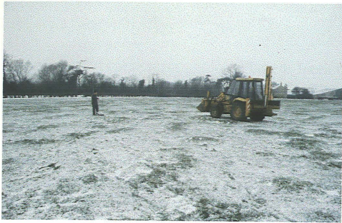
Plate 1: Starting the machining of the Trenches
