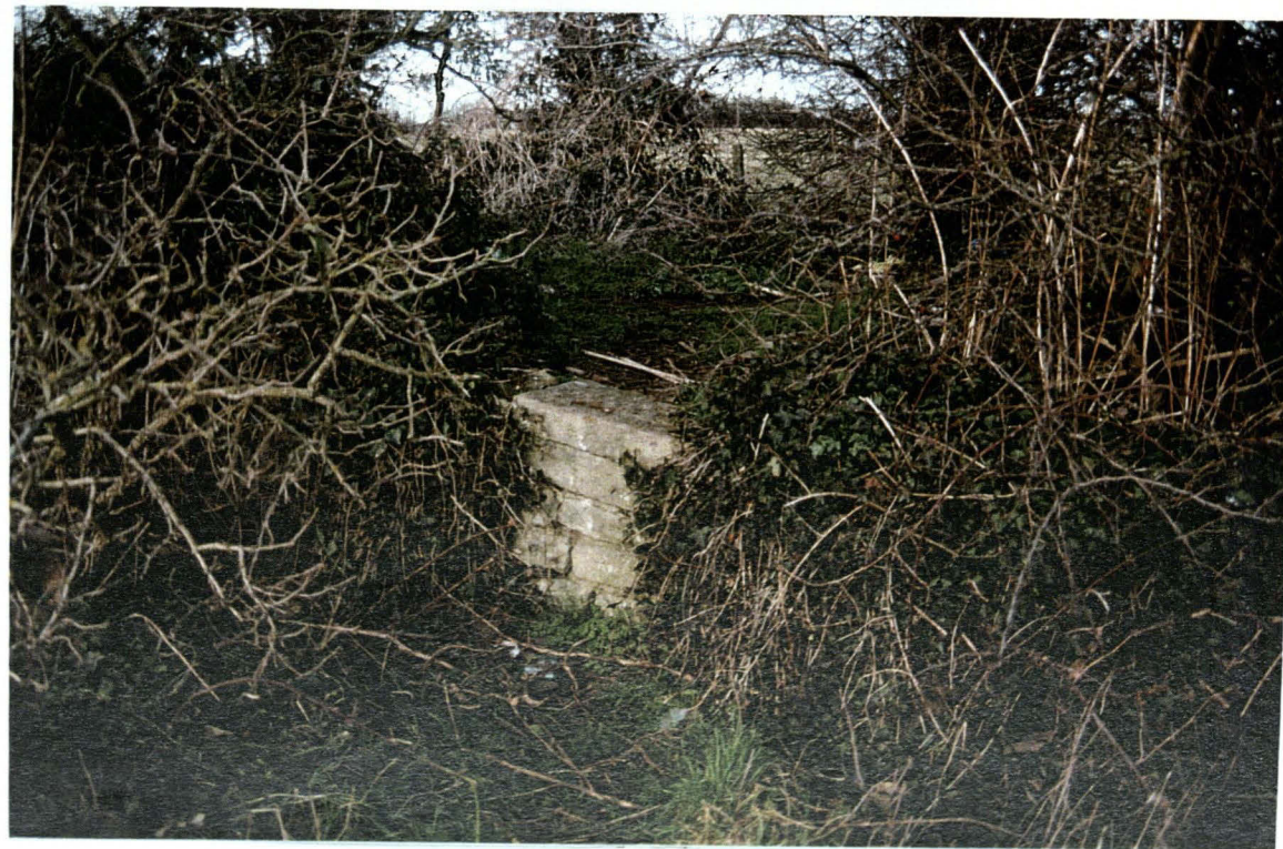
P2. The same wall, surviving above modern ground level to the east of the site
