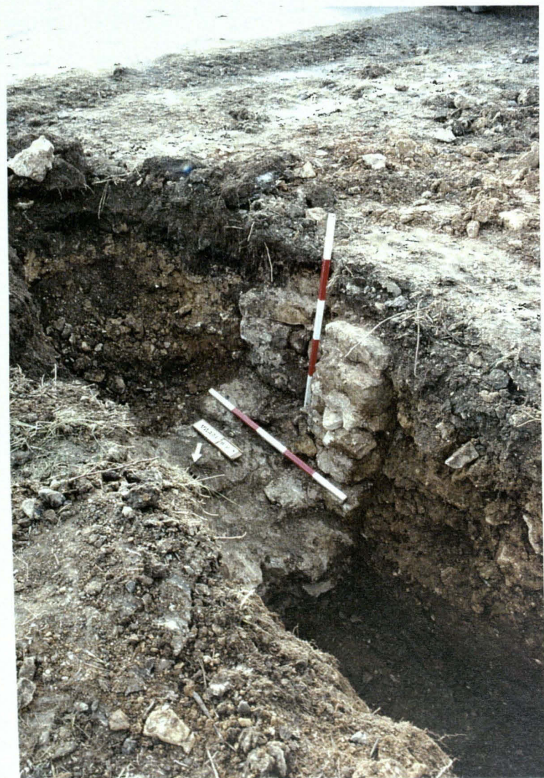
P1. Former railway boundary wall exposed in Plot 1
