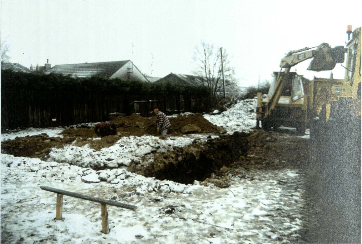
P3. General view during excavations for Plot 2, looking north-east
