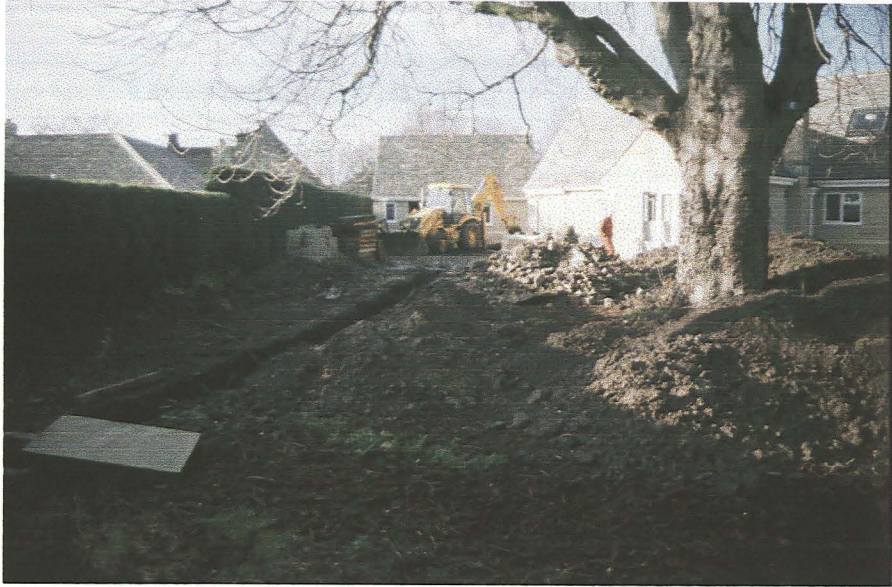
Plate 1 : General View, looking south
