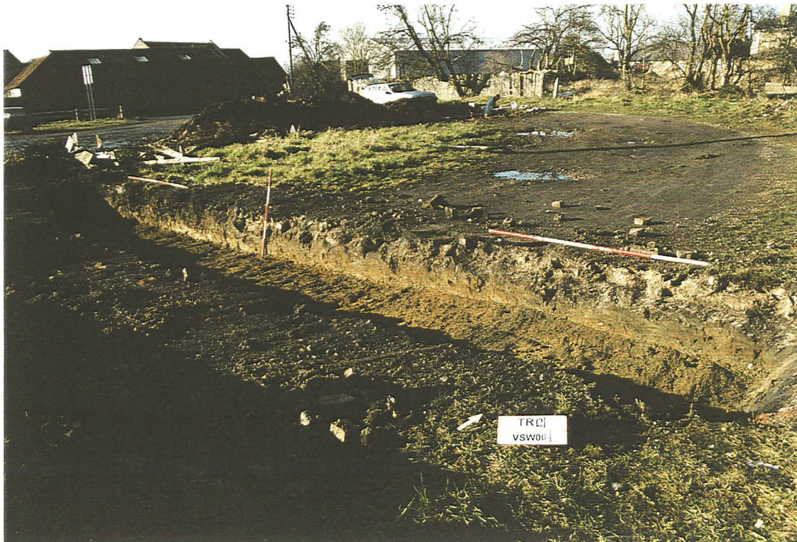
P3. General view, Trench 02, looking north-west
