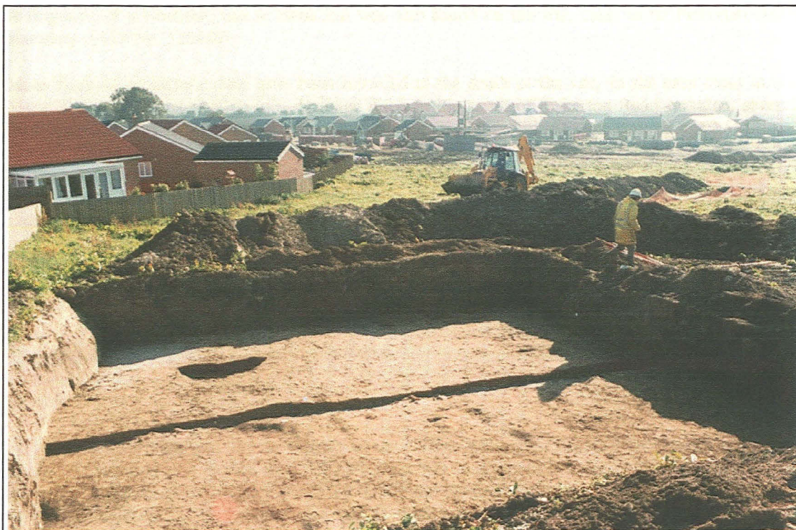
Plate 1: General view of Trench 10, looking south-east towards Trench 8.
