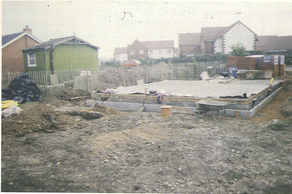
Plate 1 General site view, looking northeast.
