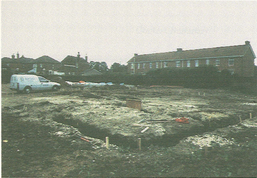
◀ Plate 1 : General Site View
