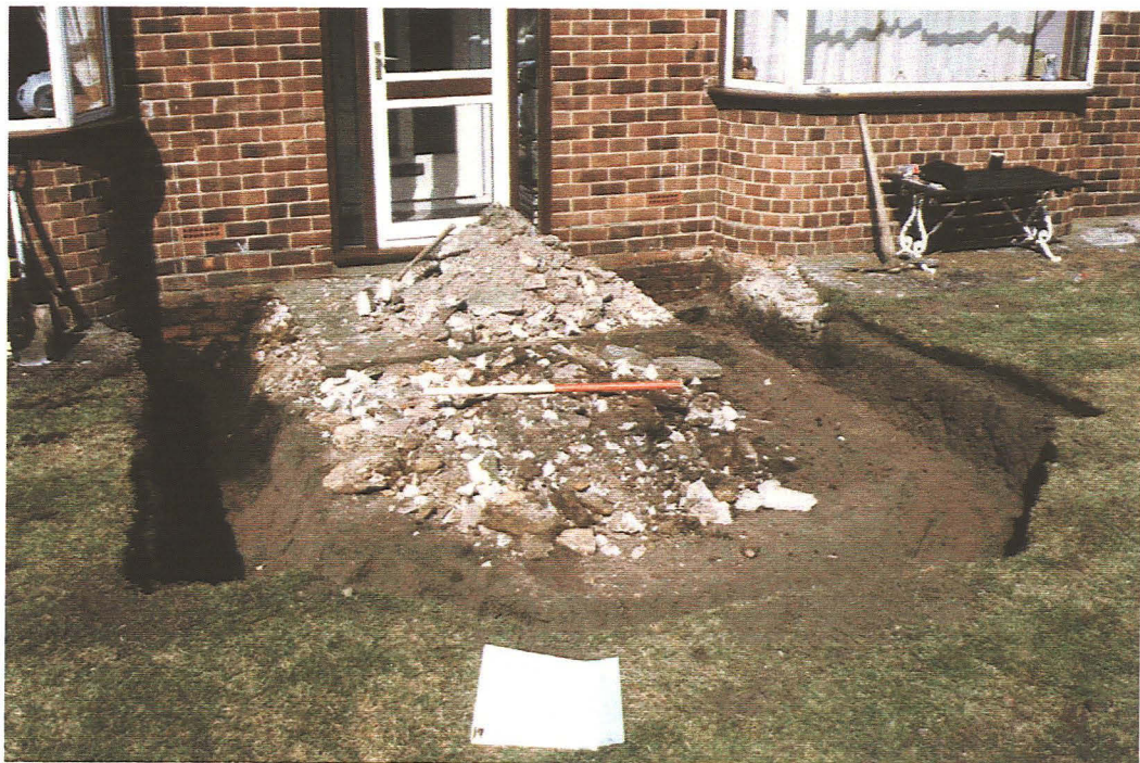
Plate 2 General view of the excavated foundation trench, looking north.
