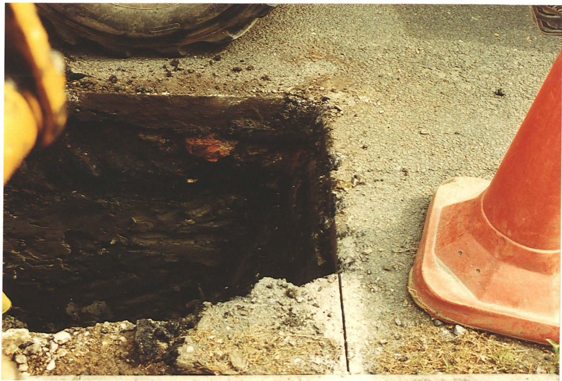
PI. 10 Post-medieval or later road foundation, Moor Lane 24, overlying brown silty clay.
