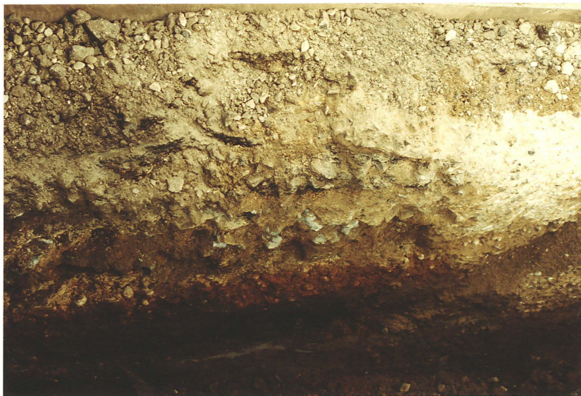
Pl. 6 Deposits below the road at 22, near Corporation Farm, showing the crushed brick layer and underlying peat.
