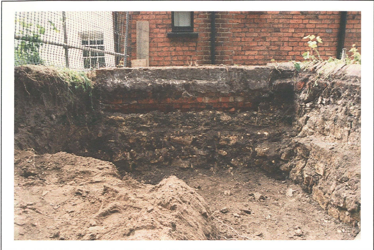
Plate 5: General view of rear of east-west retaining wall - looking south
