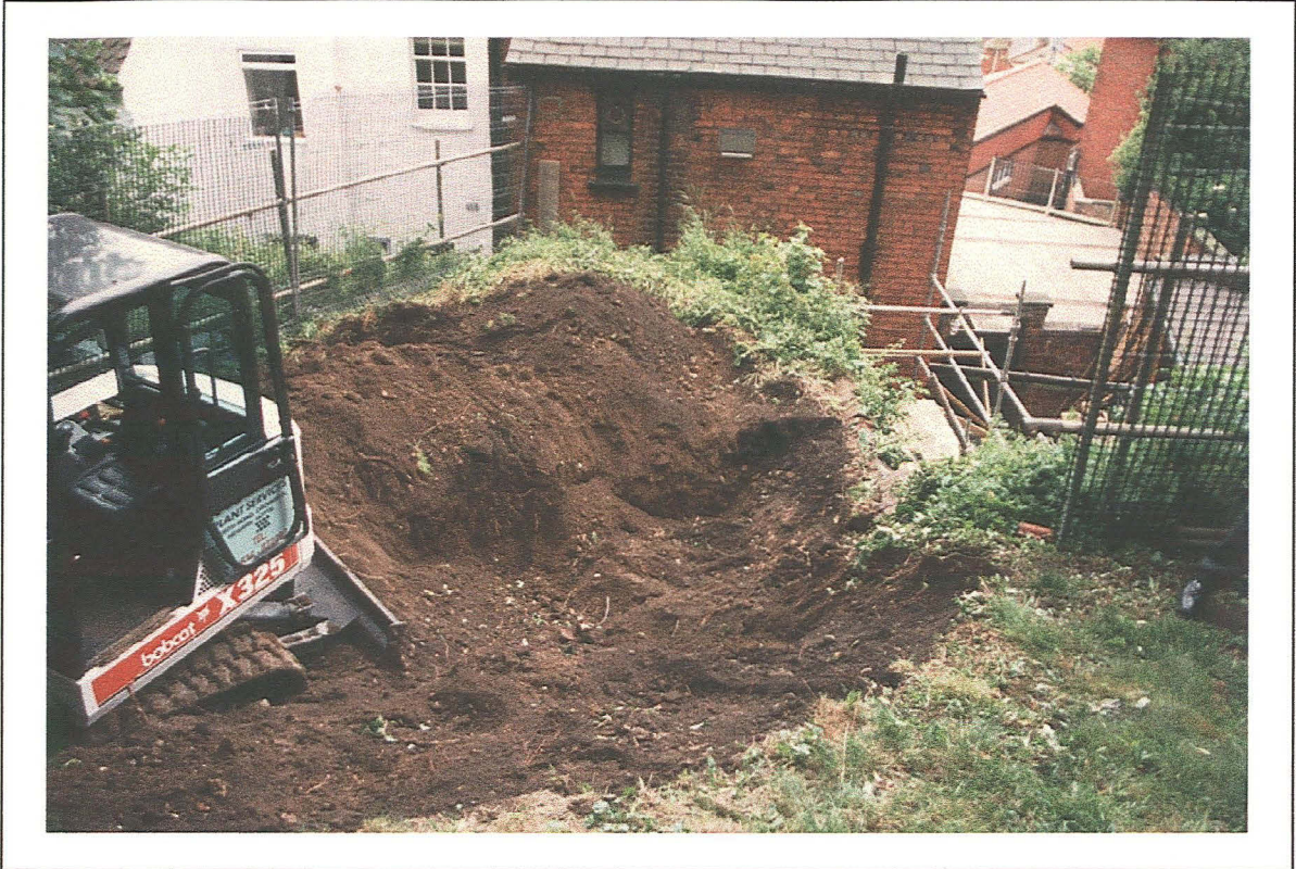
Plate 1: General view of ground level reduction underway to the rear of the retaining wall - looking south
