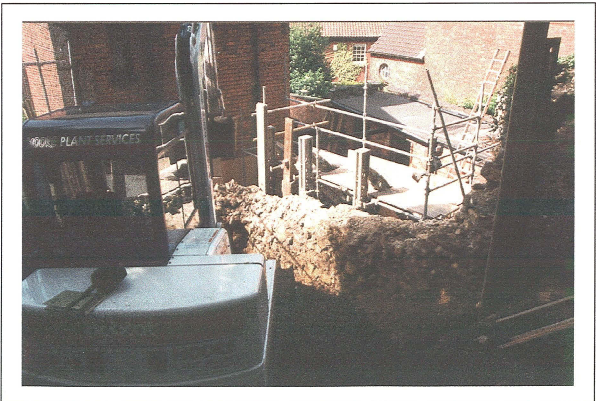
Plate 6: Overall view of lower levels of north-south retaining wall - looking south-west
