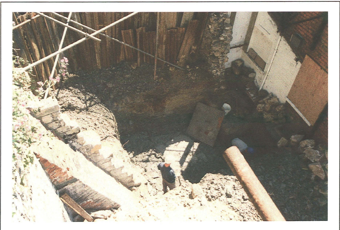
Plate 8: General view of level of new foundations - looking south-east
