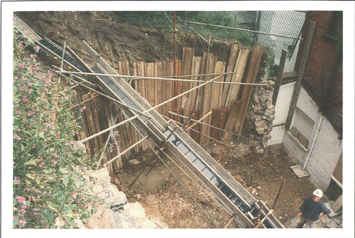
Plate 7: General view of lower levels of the excavated area - looking south-east
