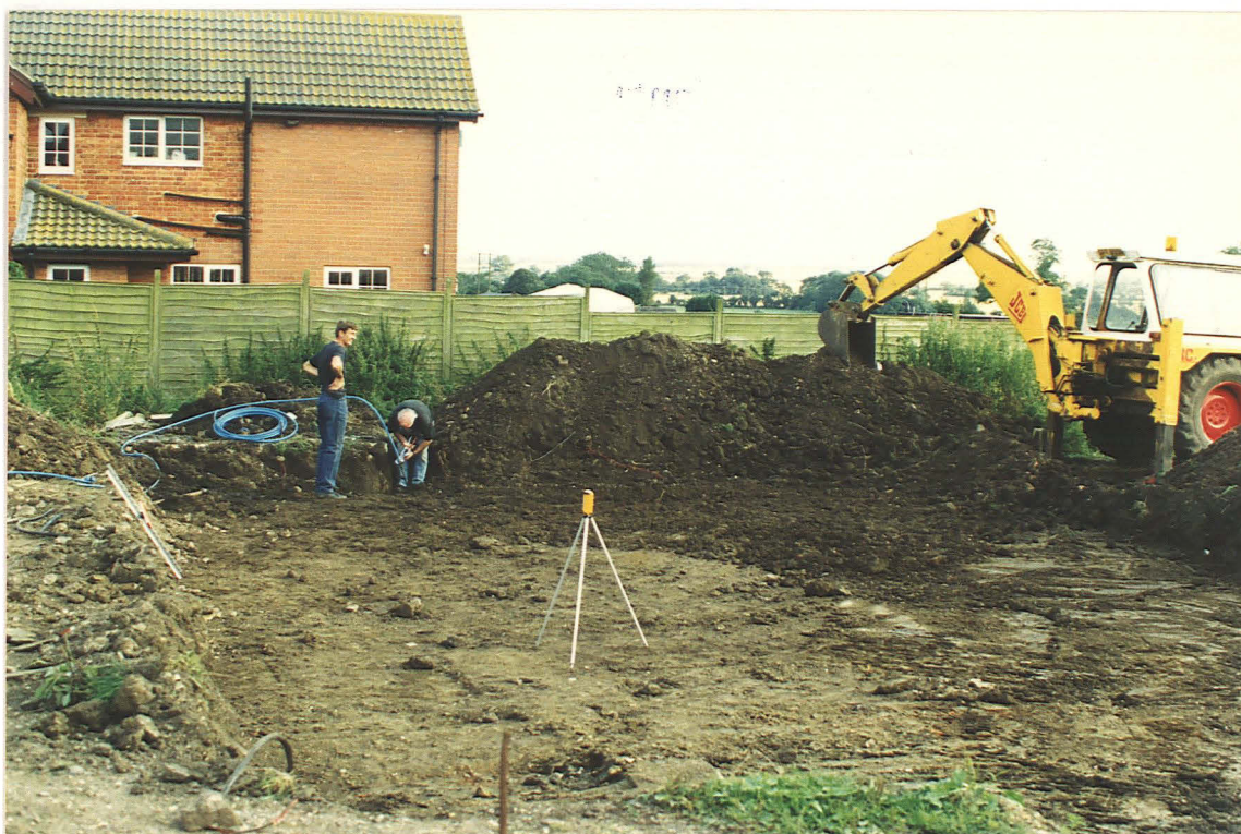
Pl. 5 Topsoil stripping in the revised house position (looking south).
