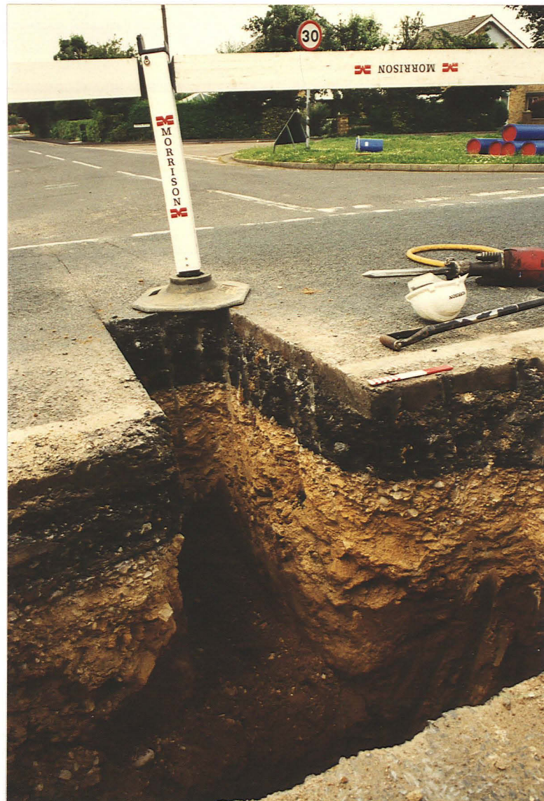
Pl. 8 Gravel metalling in the centre of Grantham Road 30, at the junction of Jensen Road (looking west).
