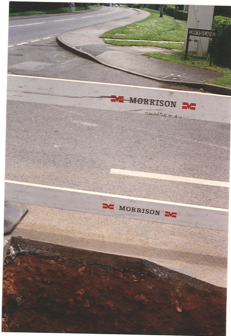
Pl. 19 Crushed brick below the tarmac surface of Davy's Lane 67 (looking south).
