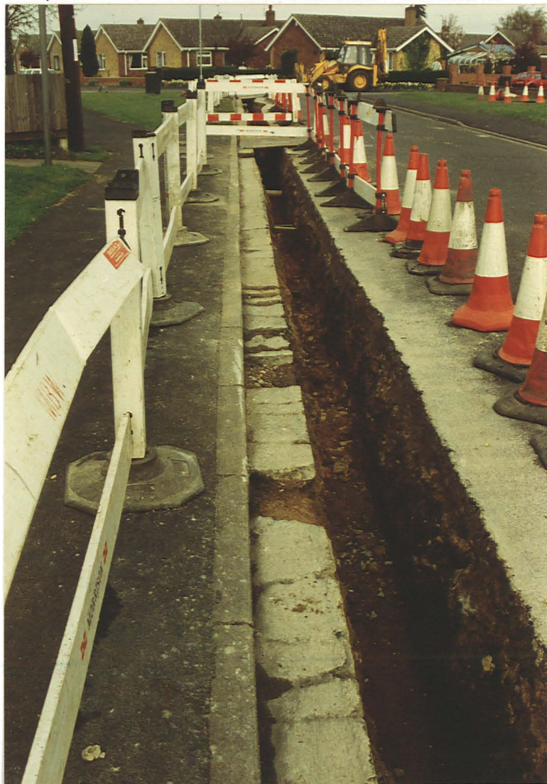
Pl. 14 Deposits exposed in the trench face, Kennedy Road 63 (looking NW). The brown soil fill of the eastern Roman roadside ditch is visible in the foreground, with the rubble road foundation behind it.
