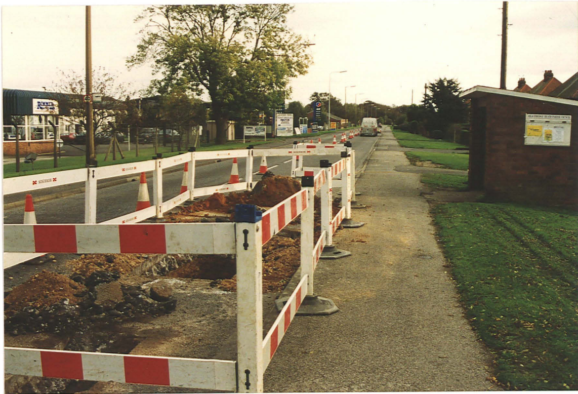
Pl. 21 Moling access holes, Sleaford Road 64 (looking SE).
