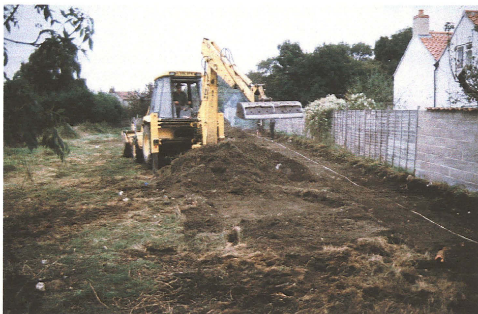
Plate 1 - General view across the development area, looking west
