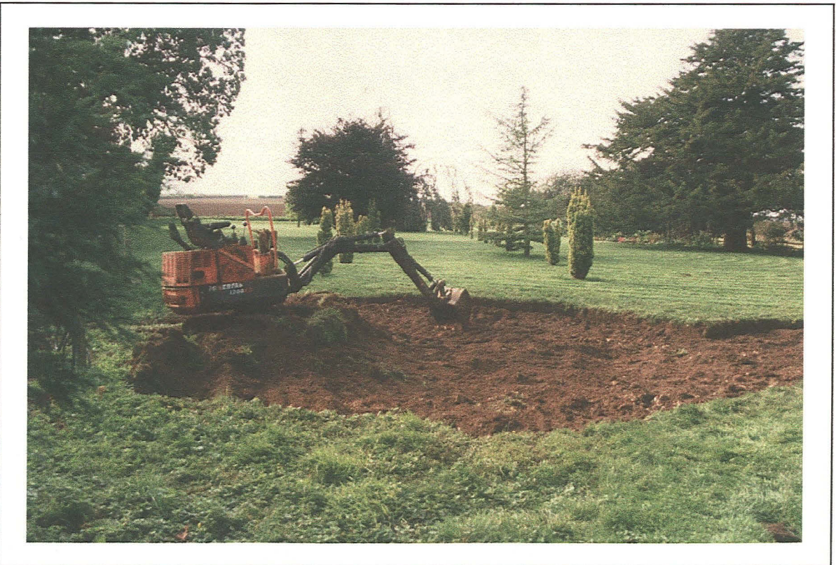
Plate 2: Overall view of groundworks in progress - looking south-west
