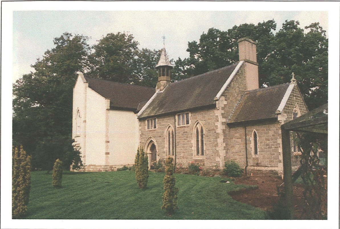
Plate 1: General view of existing property, showing added wing on left - looking north-west
