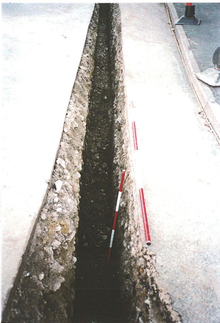
P. 4 View of excavations alongside the church, facing north
