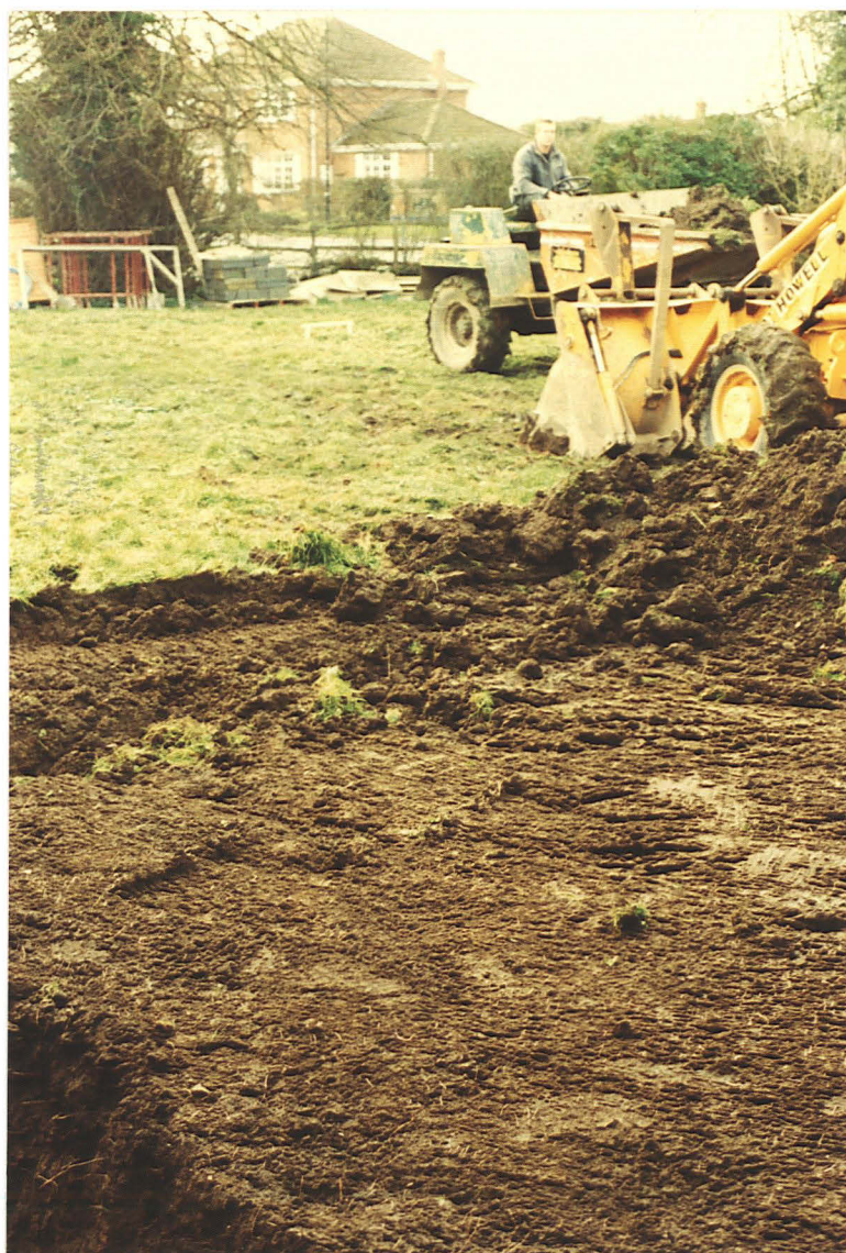
Plate 2: Stripping the development site
