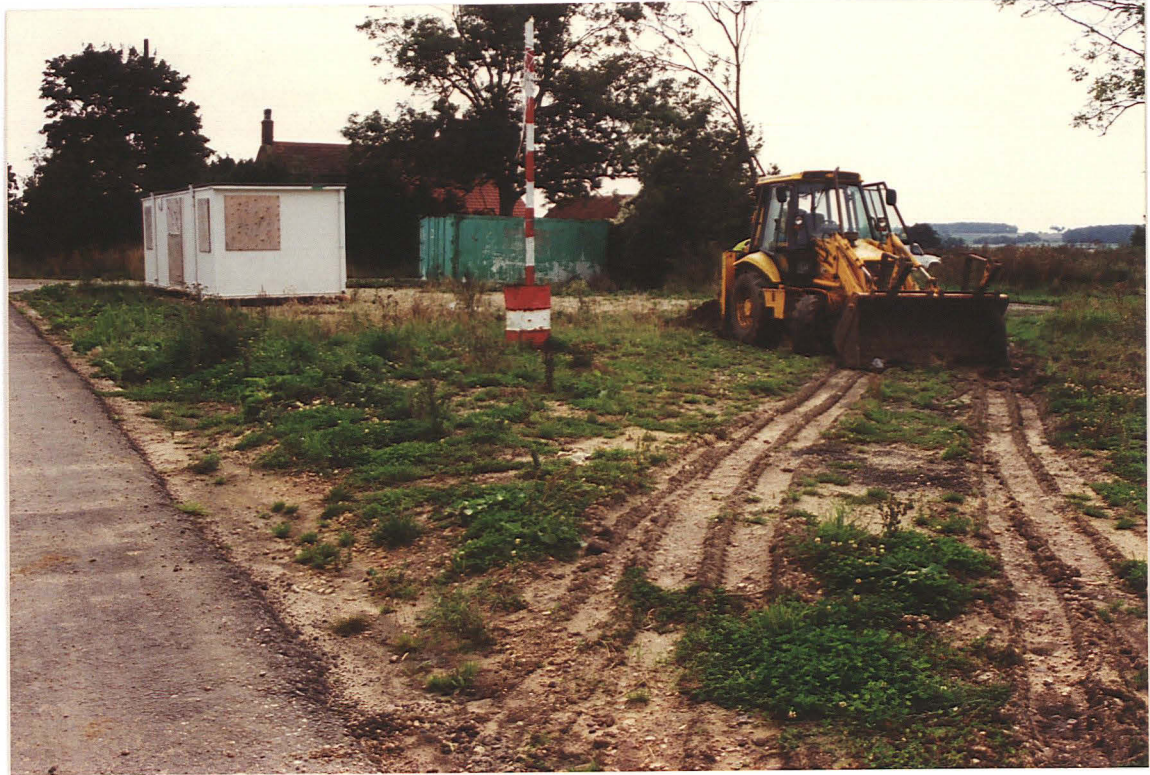
Pl. 4 Location of Geotechnical Test Pit 5 (looking south to The Farm).
