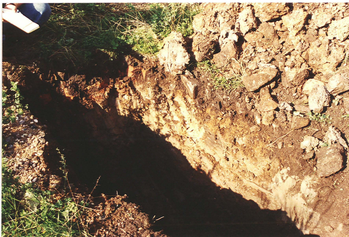
Pl. 2 Geotechnical Test Pit 2a, showing brick foundation.
