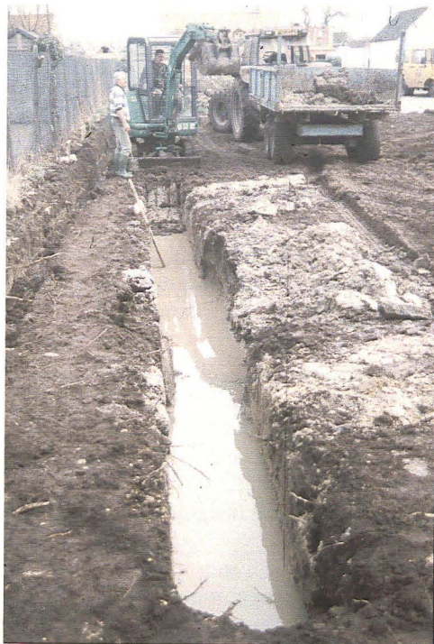
Plate 2 Excavation of footings in progress, looking east
