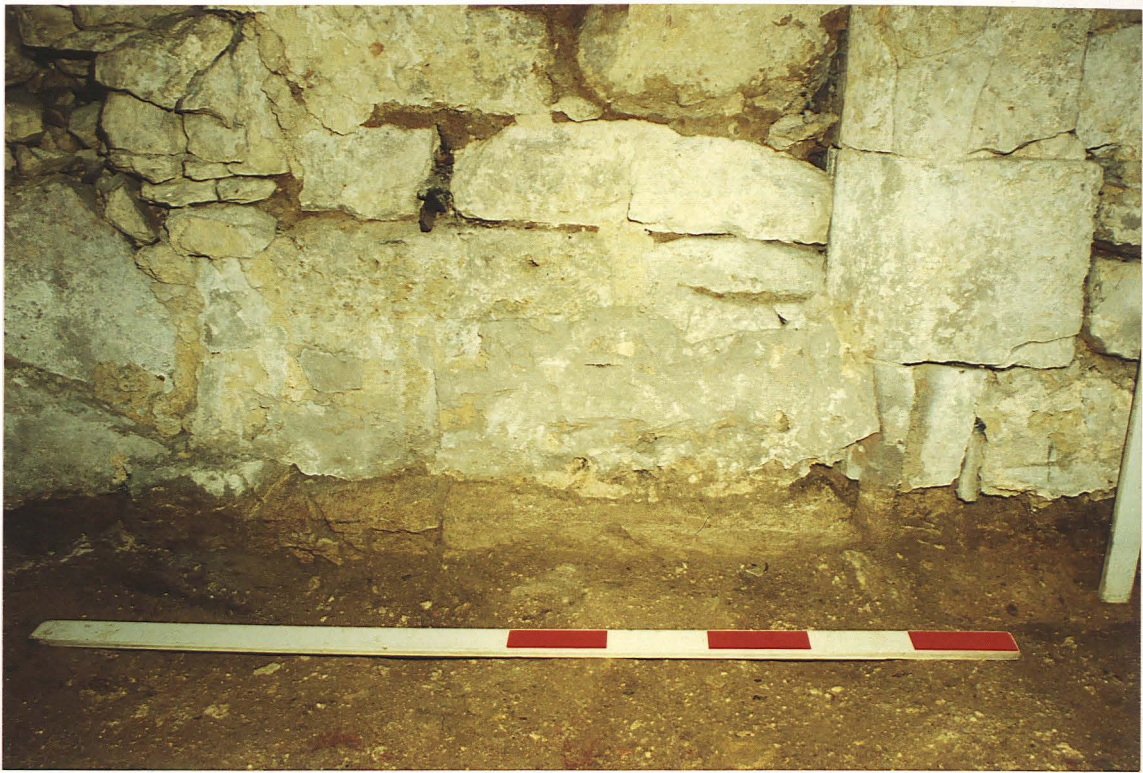
Pl. 15 Chamfered door lintel at base of Opening 2
