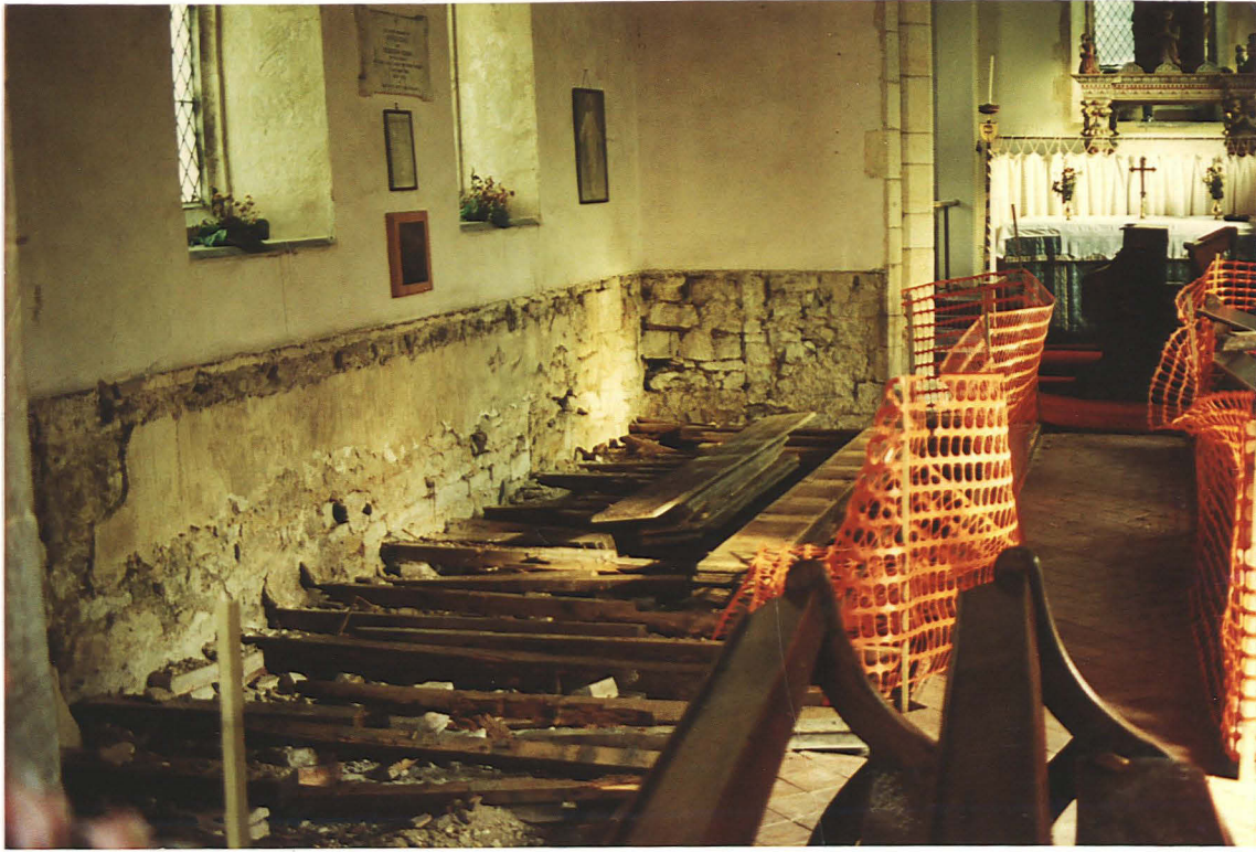
Pl. 3 The north side of the nave during the removal of the pew platform, looking east
