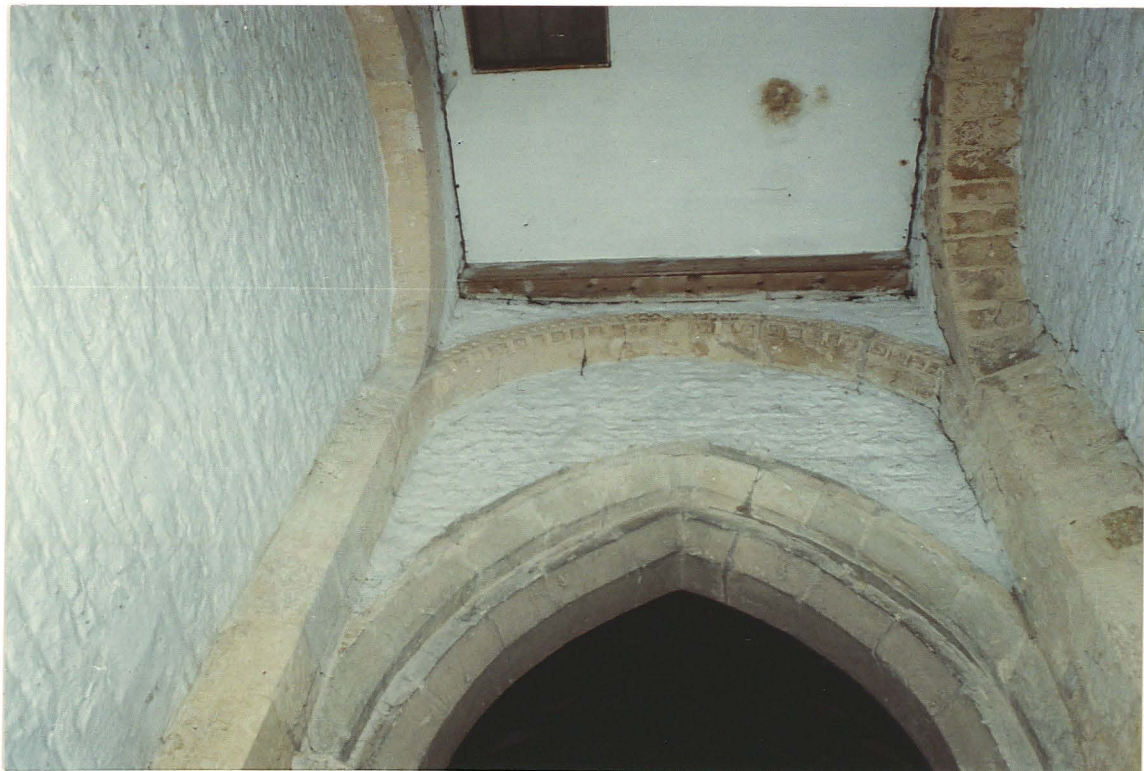
Pl. 2 The Norman tower arch and the replacement pointed arch
