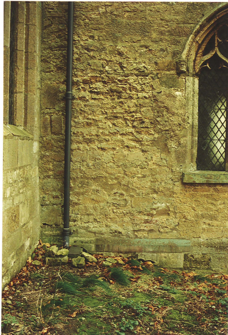
Pl. 16 Opening 2 seen in exterior wall of the church
