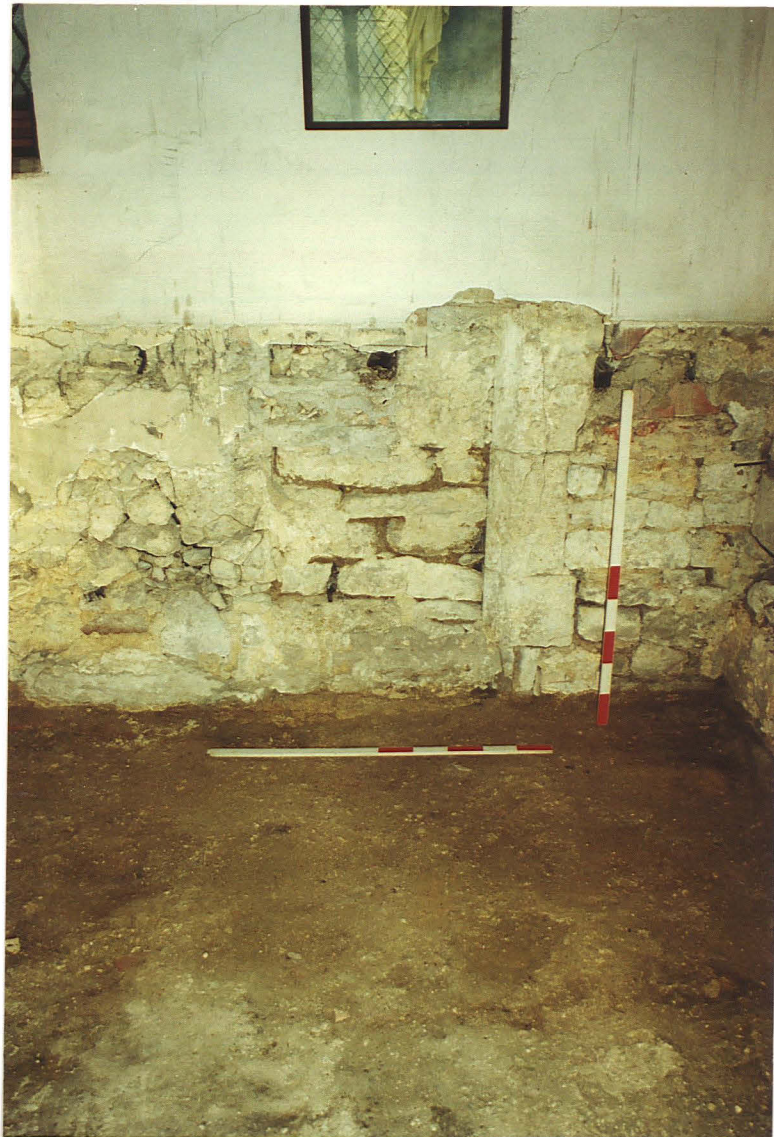
Pl. 14 Opening 2 in north wall of nave
