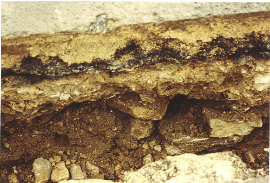
Pl. 14 Remains of stone culvert 4b, looking south.
