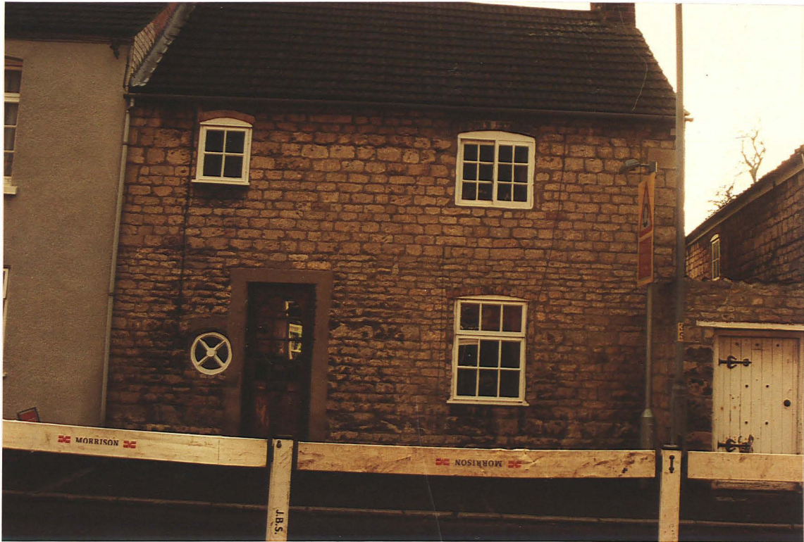
Pl. 13 The stone culvert 4b was aligned towards No. 6, Main Road (looking north).
