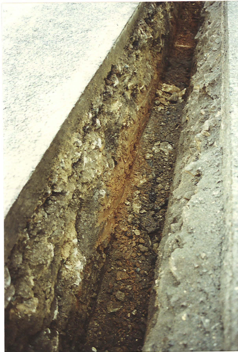
Pl. 8 Thick layer of limestone road foundation at 3, with light brown buried soil at the trench base.
