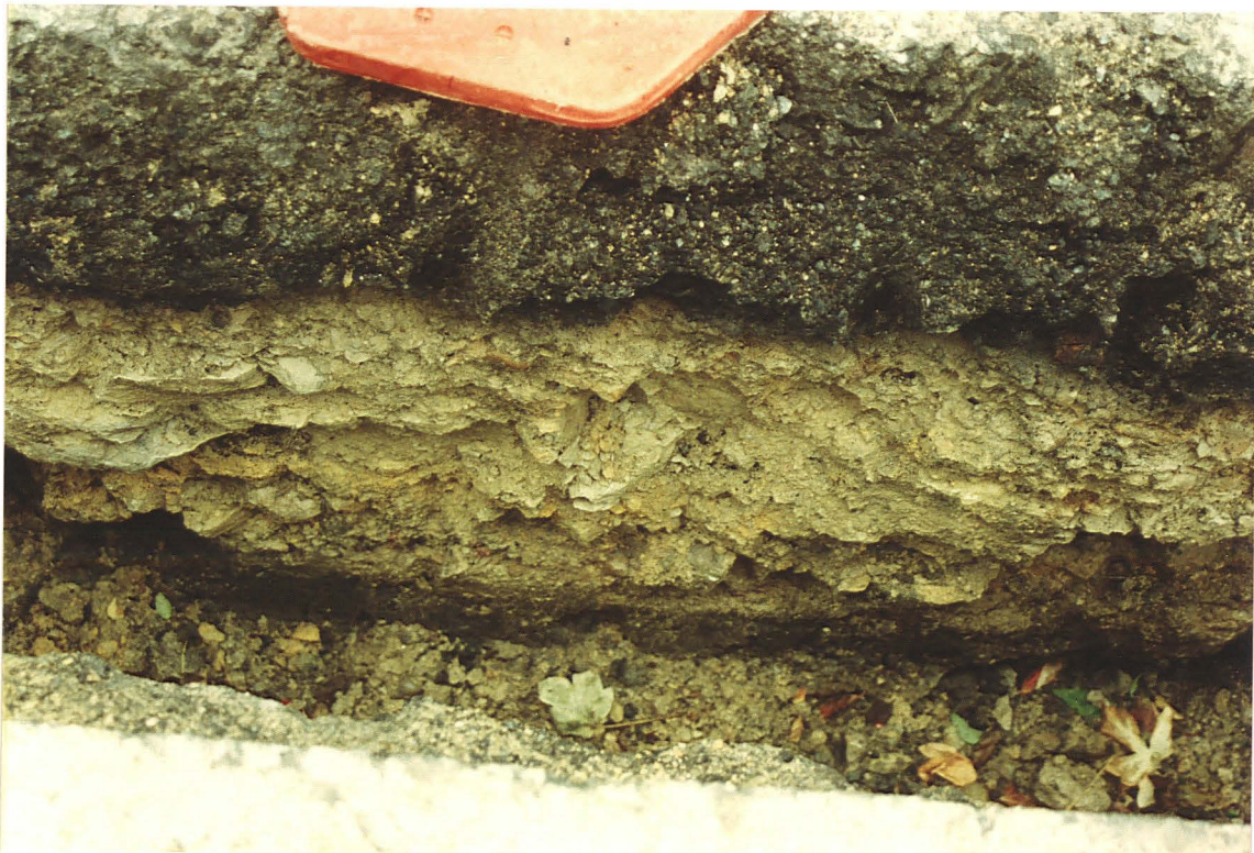
Pl. 10 Thick limestone rubble road foundation at 4a, overlying peaty material at the trench base.
