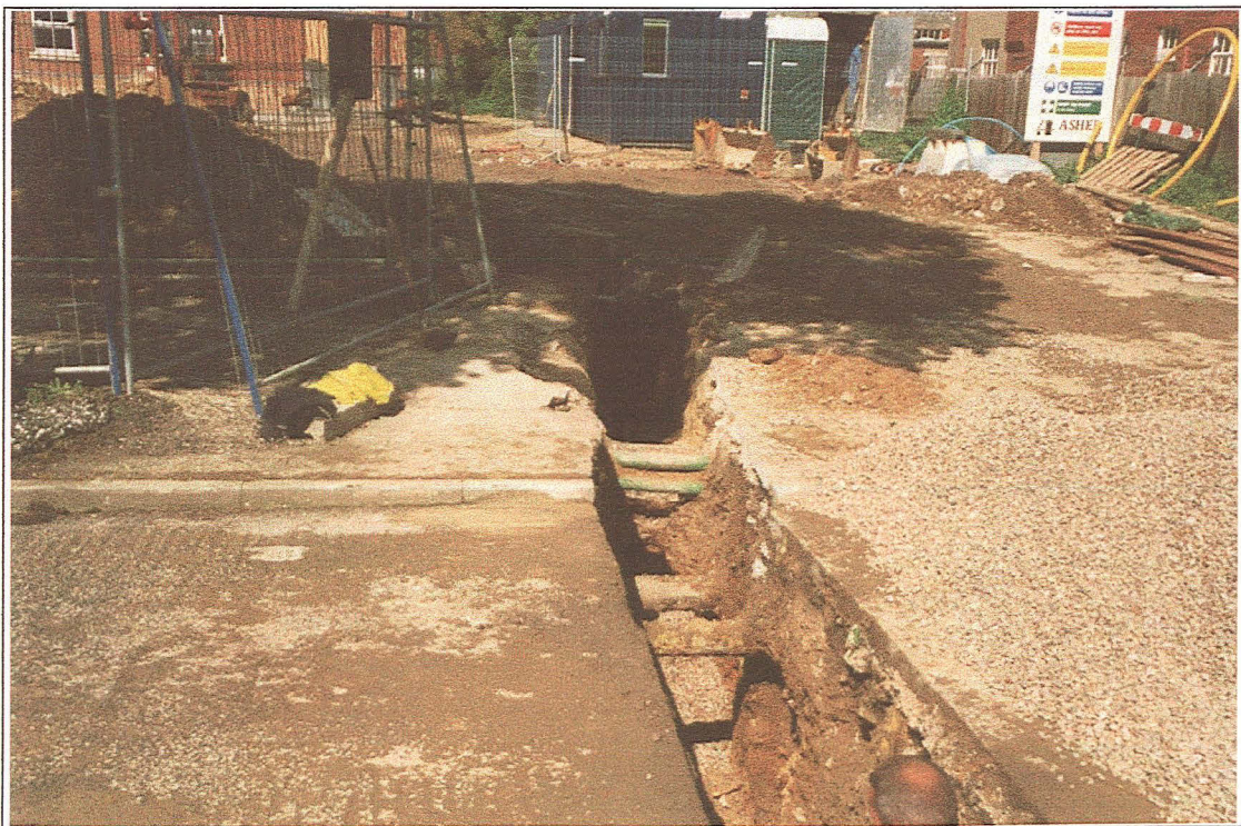
Plate 2 - Excavations in progress along Combined Services Trench into Newport (looking W)
