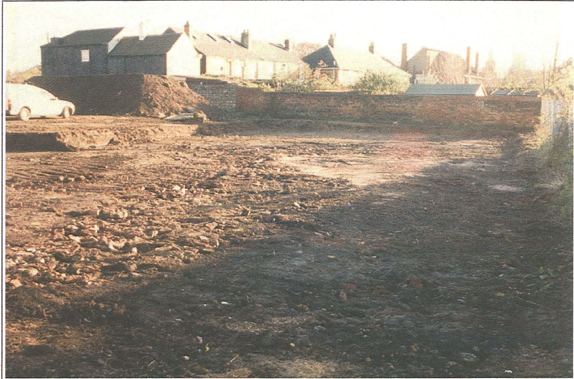
Plate 1 - Completed excavations within the footprint of the Veterinary Hospital (looking SSE)
