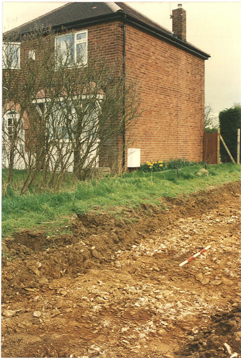
Pl. 3 Location of the Roman cremation vessel 102, found west of Ermine Street (looking NE).
