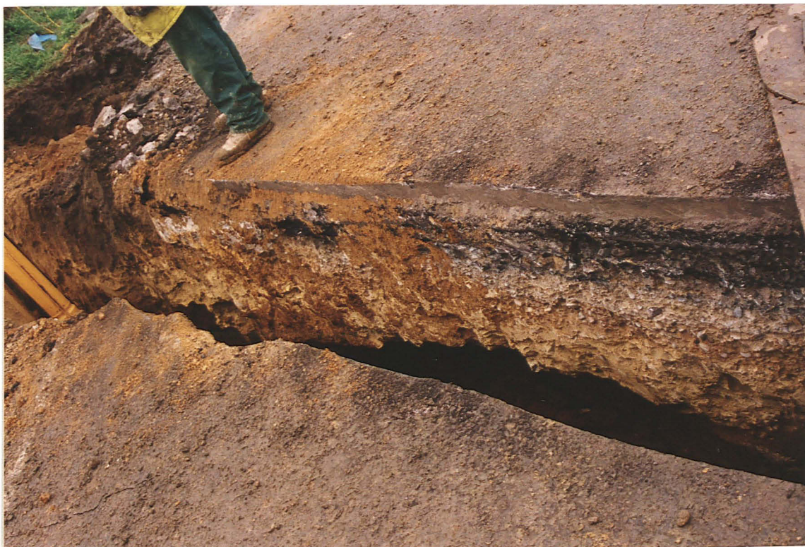
Pl. 17 The Roman gravel road surface stopped before the modern concrete road extension (left) but the crushed rock foundation extended further west into the modern verge.
