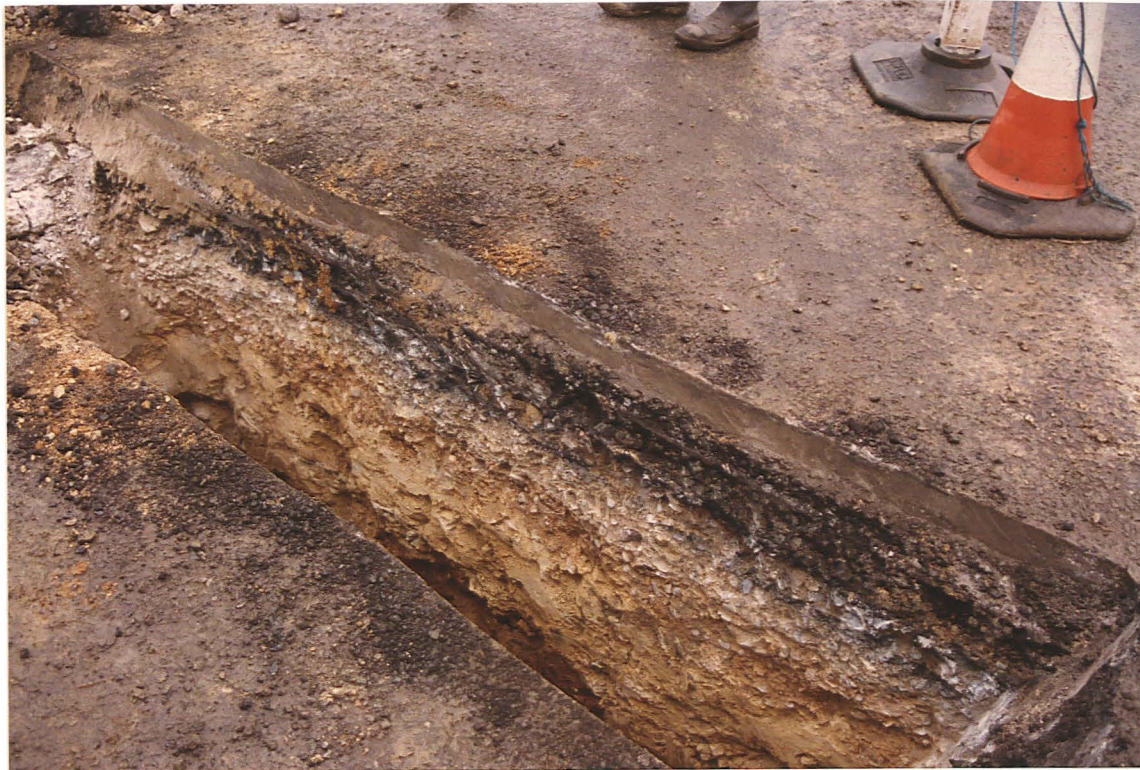
Pl. 16 Sequence of road layers below the western side of Sleaford Road. The tarmac layers overlie large angular gravel of the post-medieval road, with fine compacted rounded gravel of the Roman road surface below. That surface is bedded onto crushed limestone, with a mound of redeposited soil beneath it.
