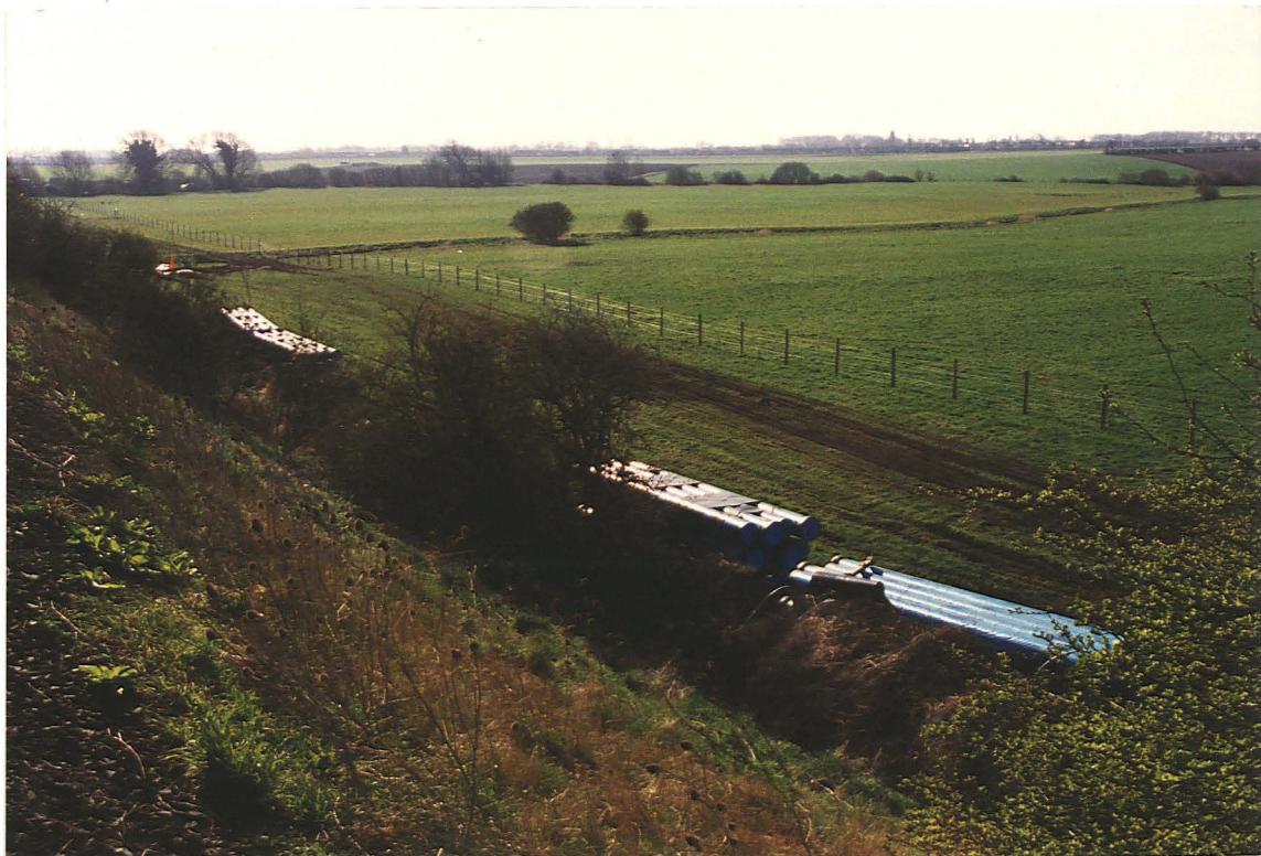
PI. 26 The southern end of the pipeline route. Dunston Pumping Station lies beyond The Beck (tall willows, far left). The fields to the north exhibit previous courses of the stream. Looking SW from the railway embankment.
